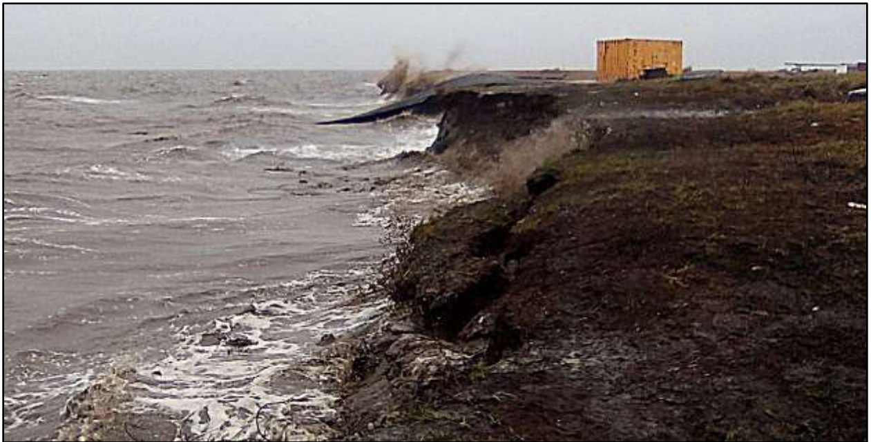
Figure 3. Storm surge actively eroding the Ninglick River bank at Newtok, October 2016 (photo courtesy of Lemay Engineering)
