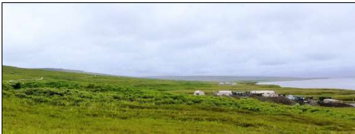
Figure 28. Mertarvik town site looking west in 2013, showing the upward slope of the land from the Ninglick River (right) towards the Nelson Island interior (left). The IRT construction camp is
