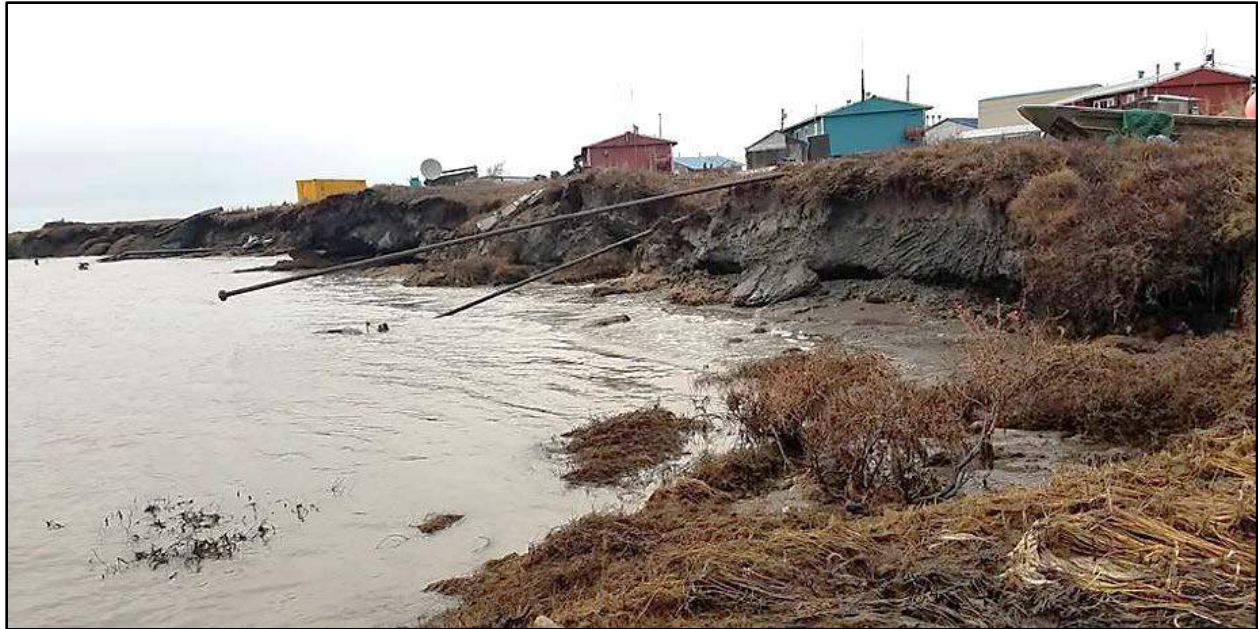
Figure 2. Breakdown of the Ninglick River bank at Newtok, October 2016 (photo courtesy of Lemay Engineering)
