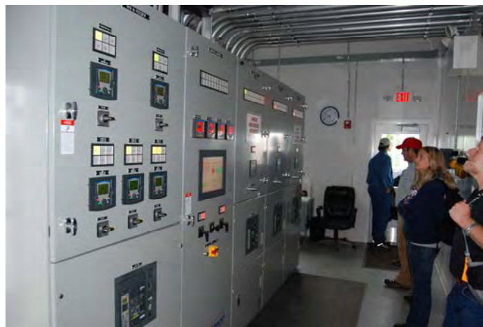
INSIDE THE KWETHLUK POWER PLANT.
