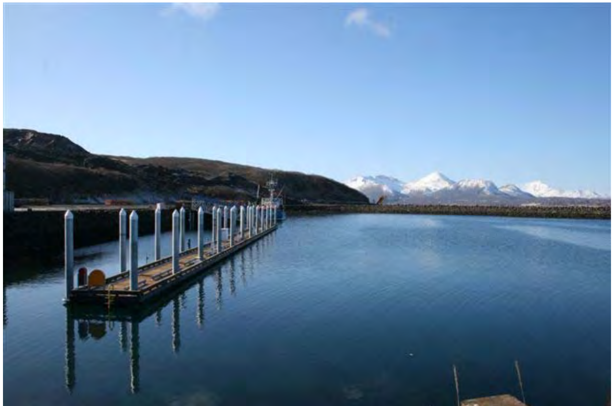
SAND POINT NEW HARBOR CONSTRUCTION
