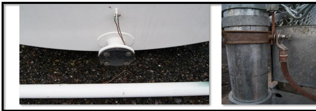
Tank Grounding Connection
