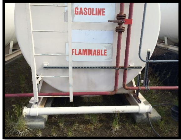
Skid Mounted Tank on a Concrete Foundation
