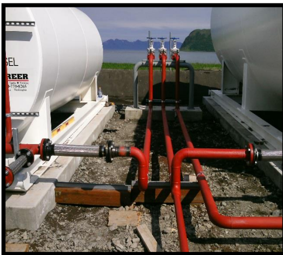
(1) (3) Welded and Flanged Joint Connections
