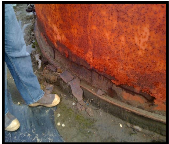
Tank Corrosion
