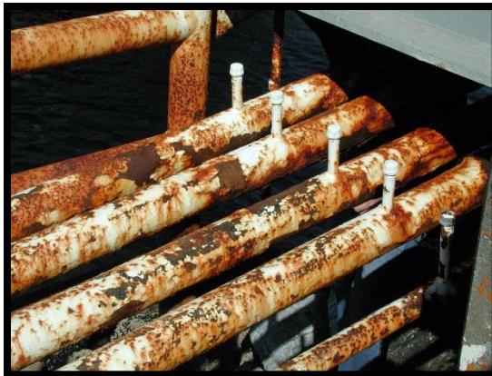
Pipe Corrosion
