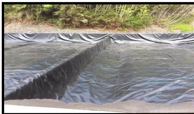
Tank Farm Liner Installation
