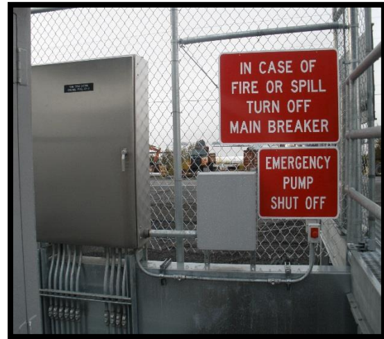
Emergency Shut-off Switch
