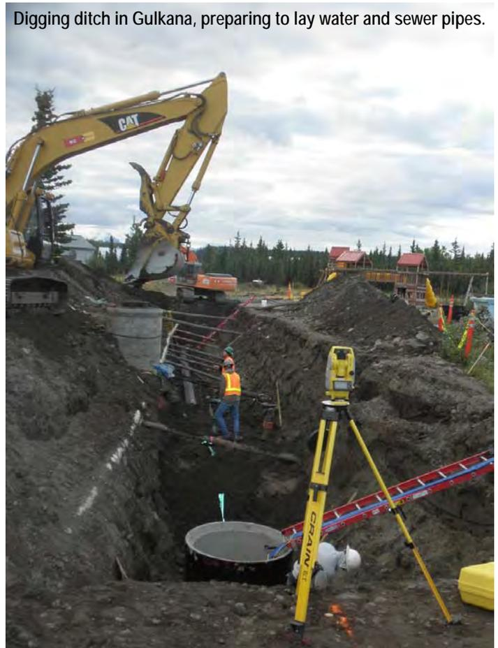
Digging ditch in Gulkana, preparing to lay water and sewer pipes.
