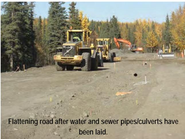
Flattening road after water and sewer pipes/culverts have been laid.
