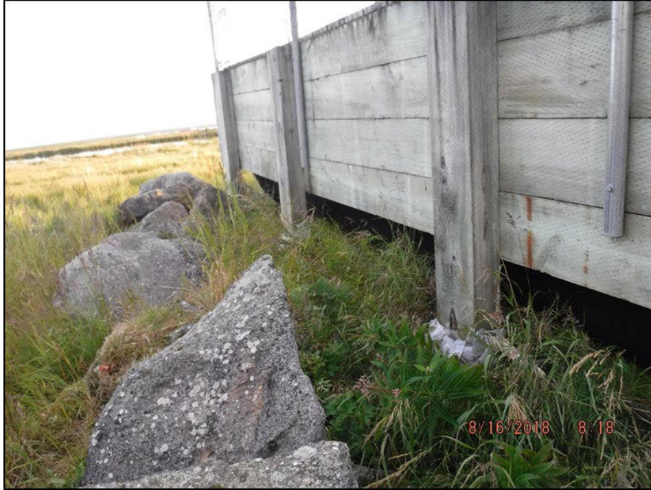
Photograph 21: Northwest corner of tank farm containment. Construction drawings show that the bottom timber should lie on the ground surface. Note stretched geotextile and liner material.
