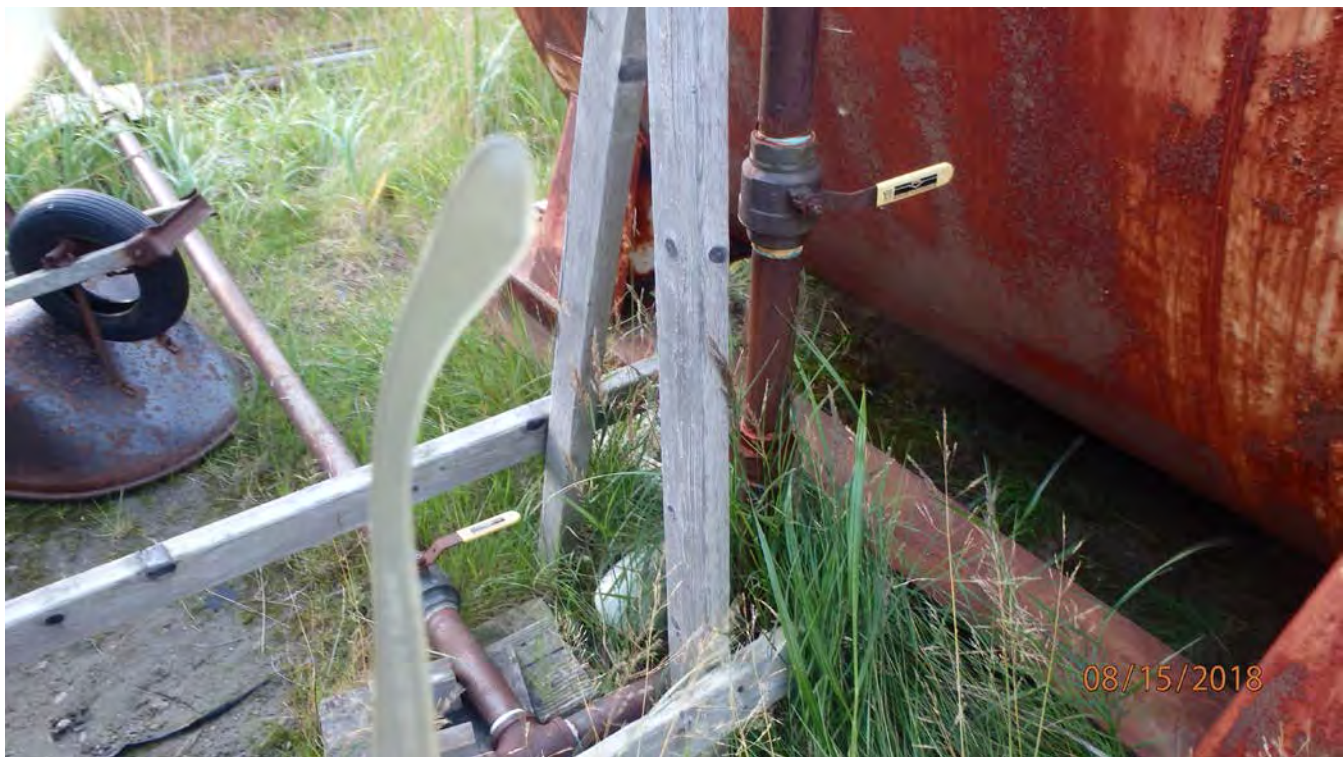
Brass Valves on piping to winter dispenser and council tank.
