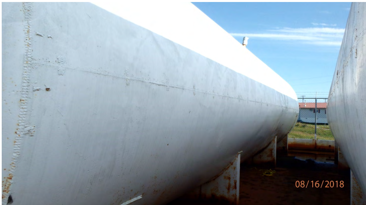
FIGURE 8: NON-STANDARD SHELL CONSTRUCTION FOR TANK 12. LONG SEAM WELDS ONLY, SHELL IS FABRICATED FROM 6 PLATES MEASURING 5.25 FEET BY 42.5 FEET LONG.
