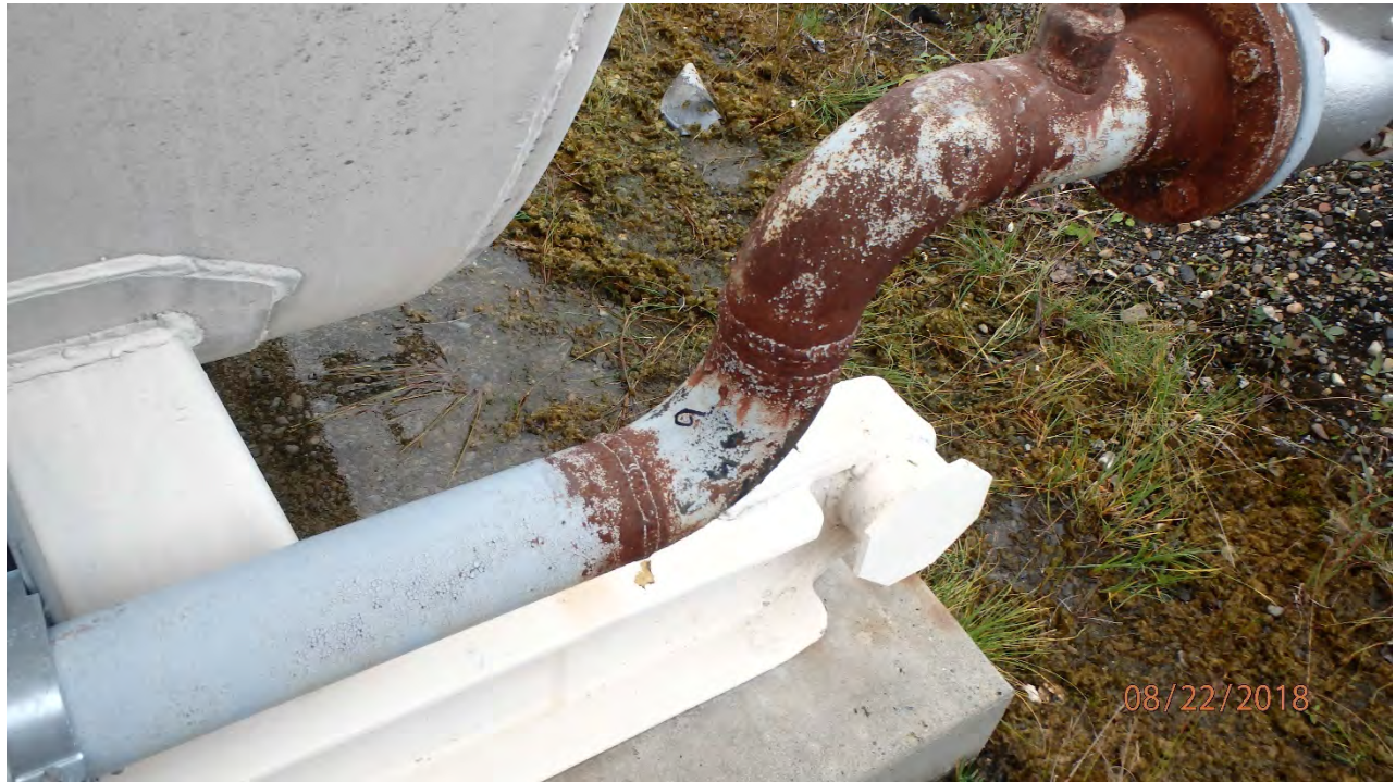
FIGURE 16: TYPICAL CONDITION FOR WELD ZONES, FITTINGS AND FLANGES ON THE DIESEL PIPING.
