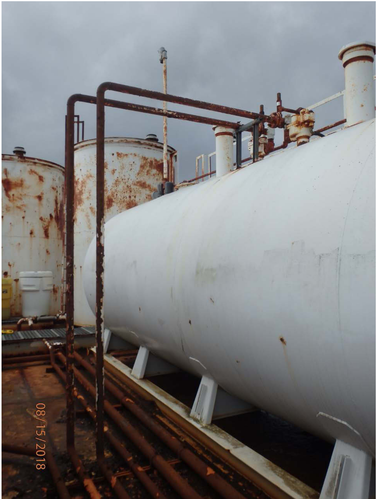
Typical tankfarm piping condition showing complete coating failure and generalized corrosion.
