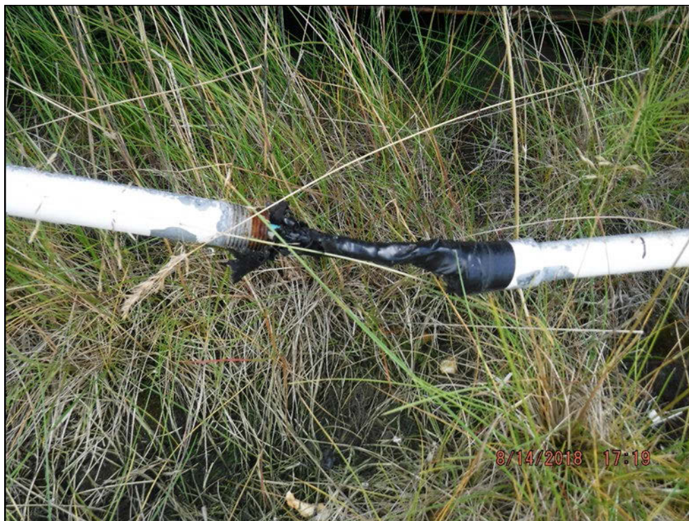
Photograph 9: Broken security light electrical conduit.
