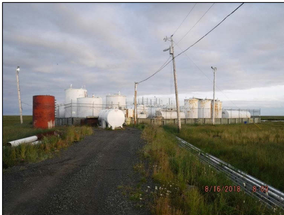
Photograph 2: Looking west at the Chefnorak Bulk Fuel Facility. Note leaning timber utility poles.
