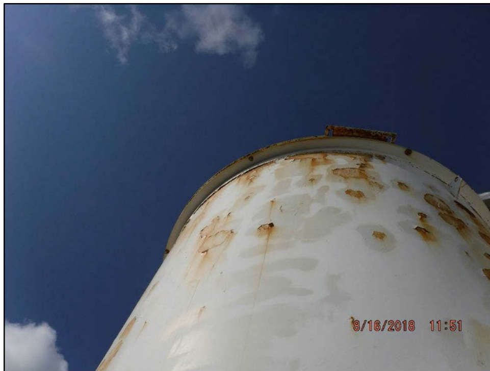
Photograph 12: Looking up at Tank #12. Note the caulking used to seal gap along tank rim.
