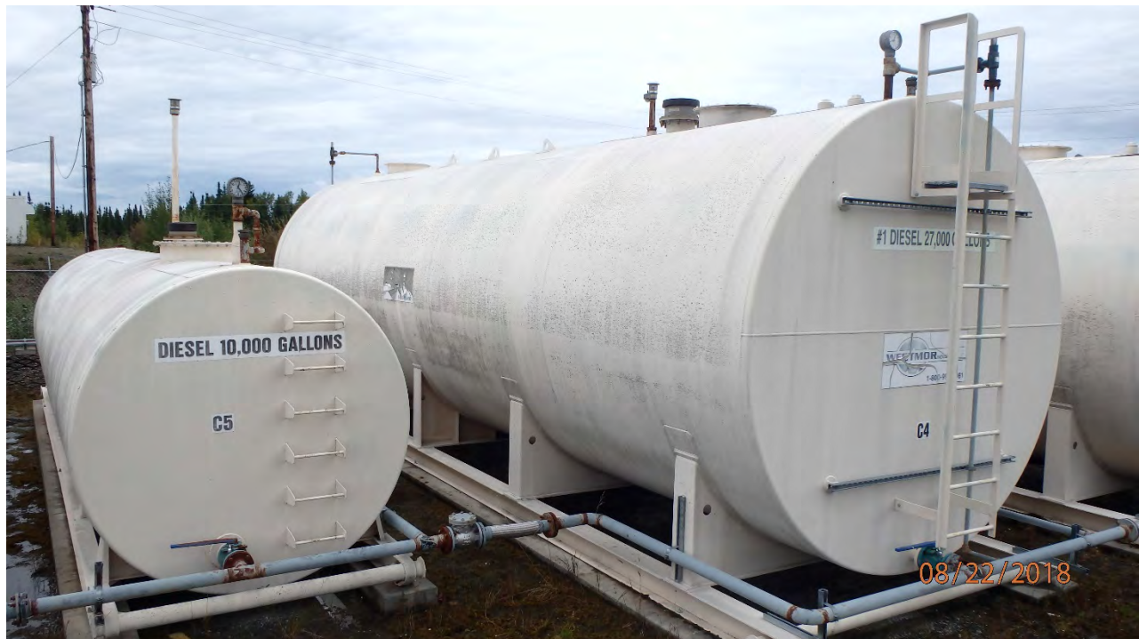
FIGURE 2: NEW DIESEL TANK (C4)
