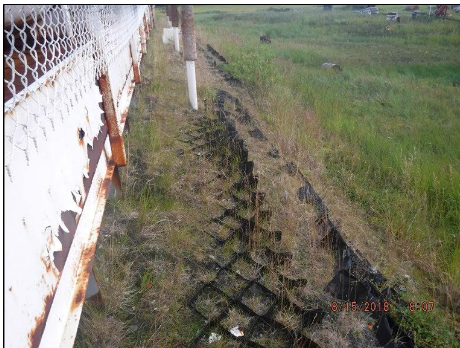
Photograph 12: Looking north along east edge of containment. Typical condition of pad edge with exposed cellular confinement.
