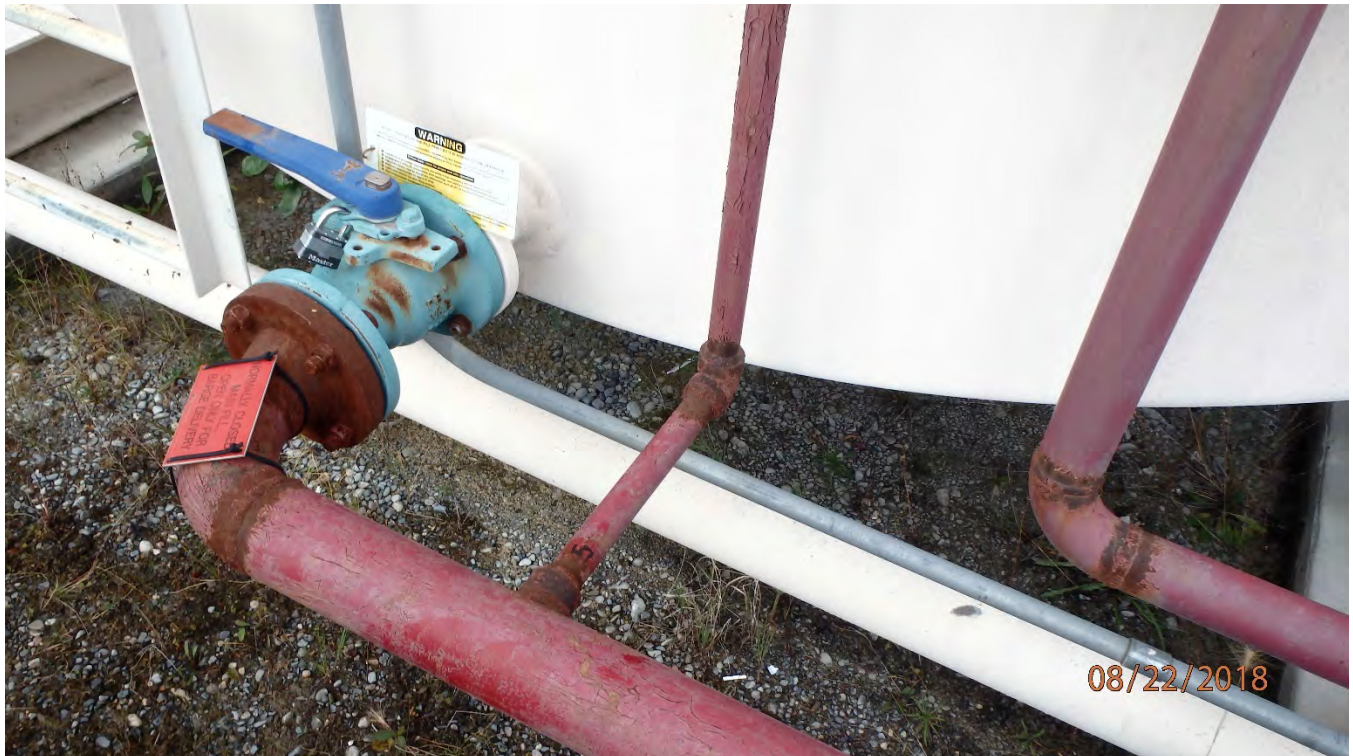
FIGURE 17: TYPICAL CONDITION FOR WELD ZONES, FITTINGS AND FLANGES ON THE GASOLINE PIPING.
