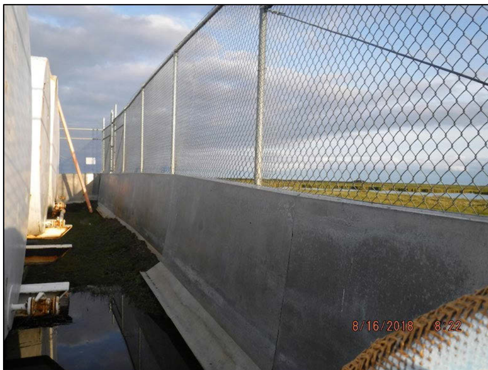
Photograph 18: Looking south along the west wall. Note where fill has subsided below the previously buried sheet metal wing.
