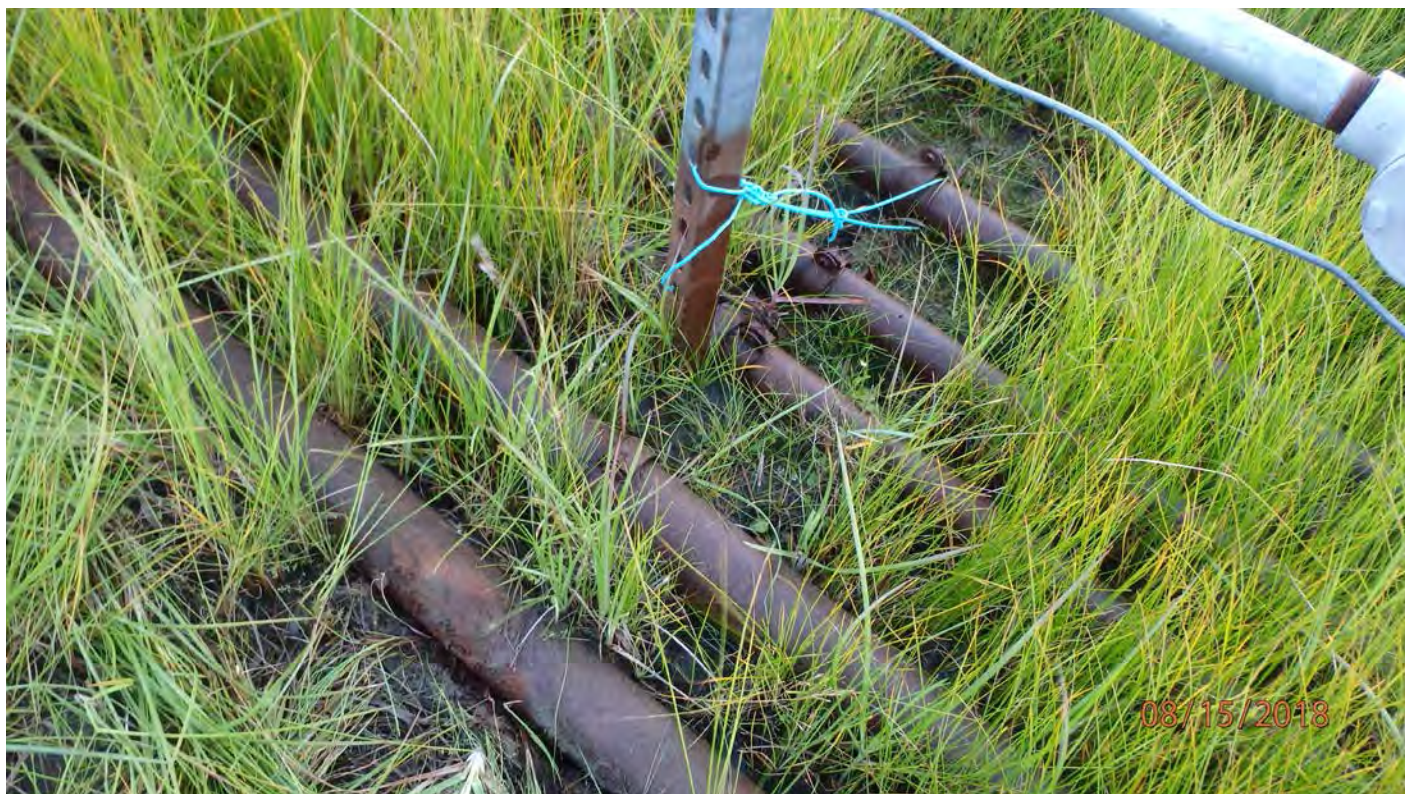
Low piping from marine header to tank farm. ~190 feet of piping is in contact with the ground or submerged for part of the year.
