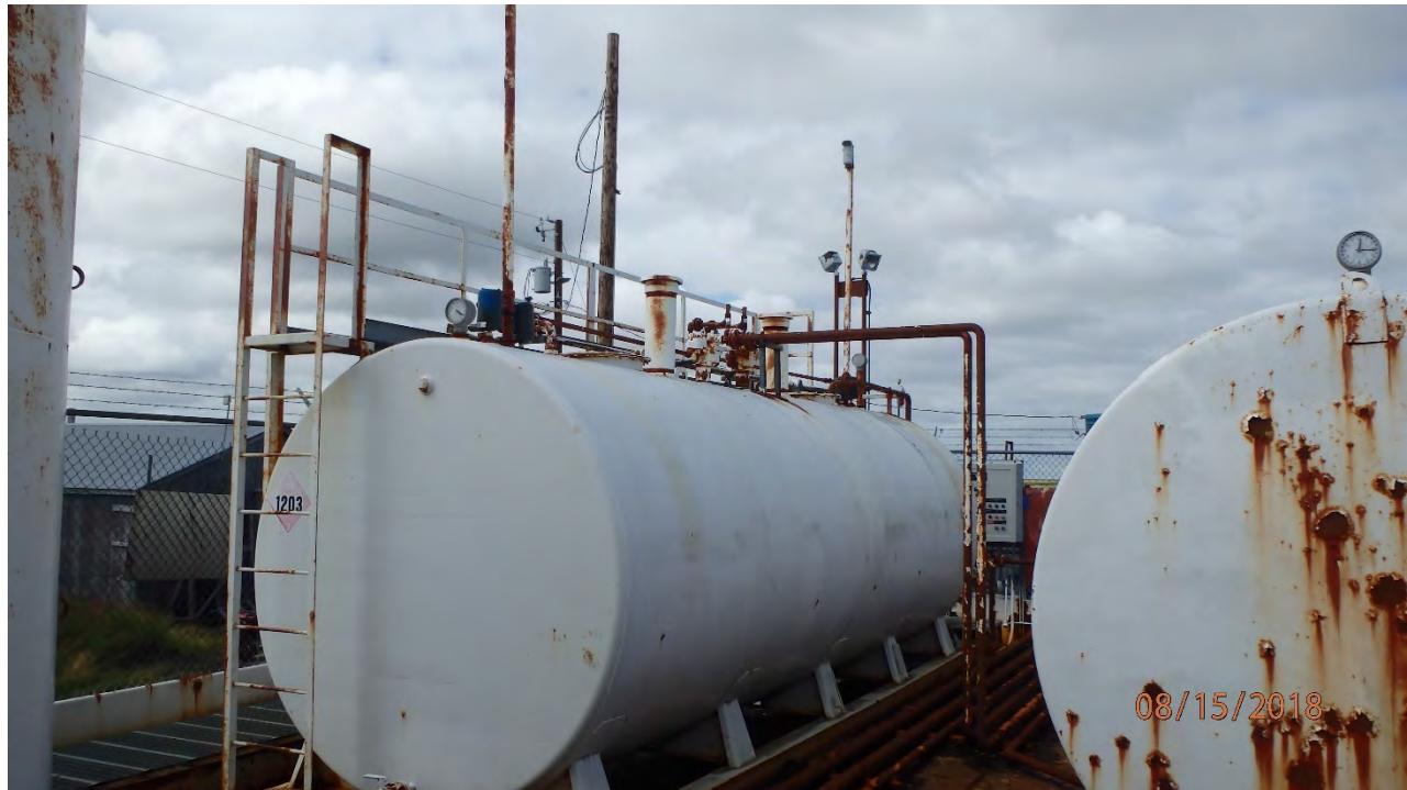
FIGURE 1: TANK 1, TWO COMPARTMENT DISPENSING TANK. UL LISTED
