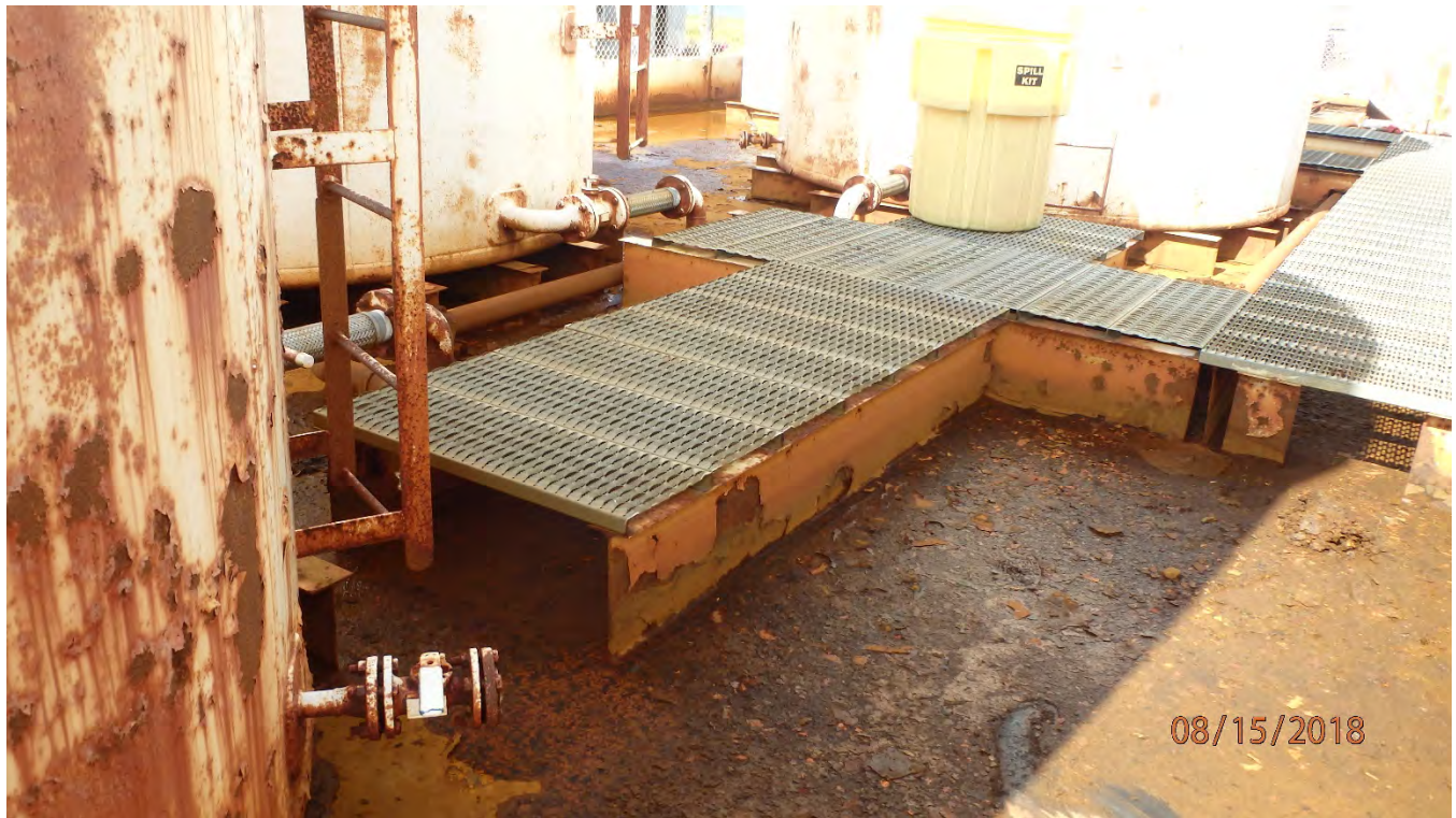
FIGURE 24: STEEL CONTAINMENT GENERAL CONDITION, NOTE FAILING COATINGS AND RUST/DEBRIS BUILD-UP.
