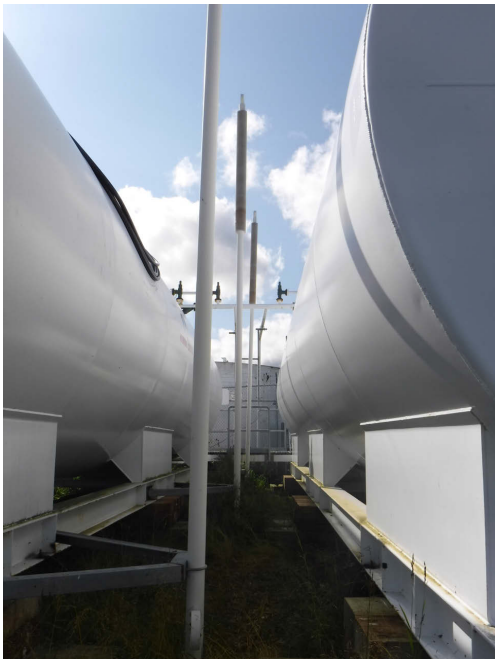
Figure 13: Thermosyphons between the tanks
