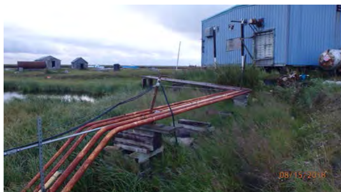
Same pipe during 2018 inspection showing complete coating failure.
