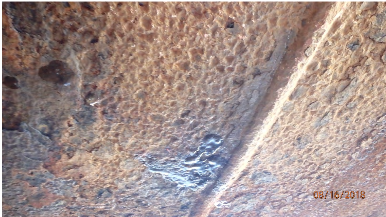
FIGURE 5: TANK 4 TYPICAL BOTTOM CONDITION WITH EXTERNAL PITTING TO 80 MILS DEEP.
