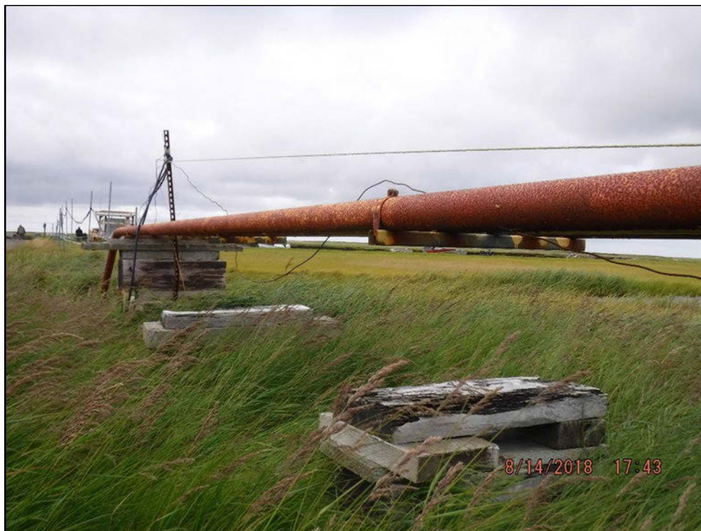
Photograph 11: Unsupported pipe run. Note partial cribbing.
