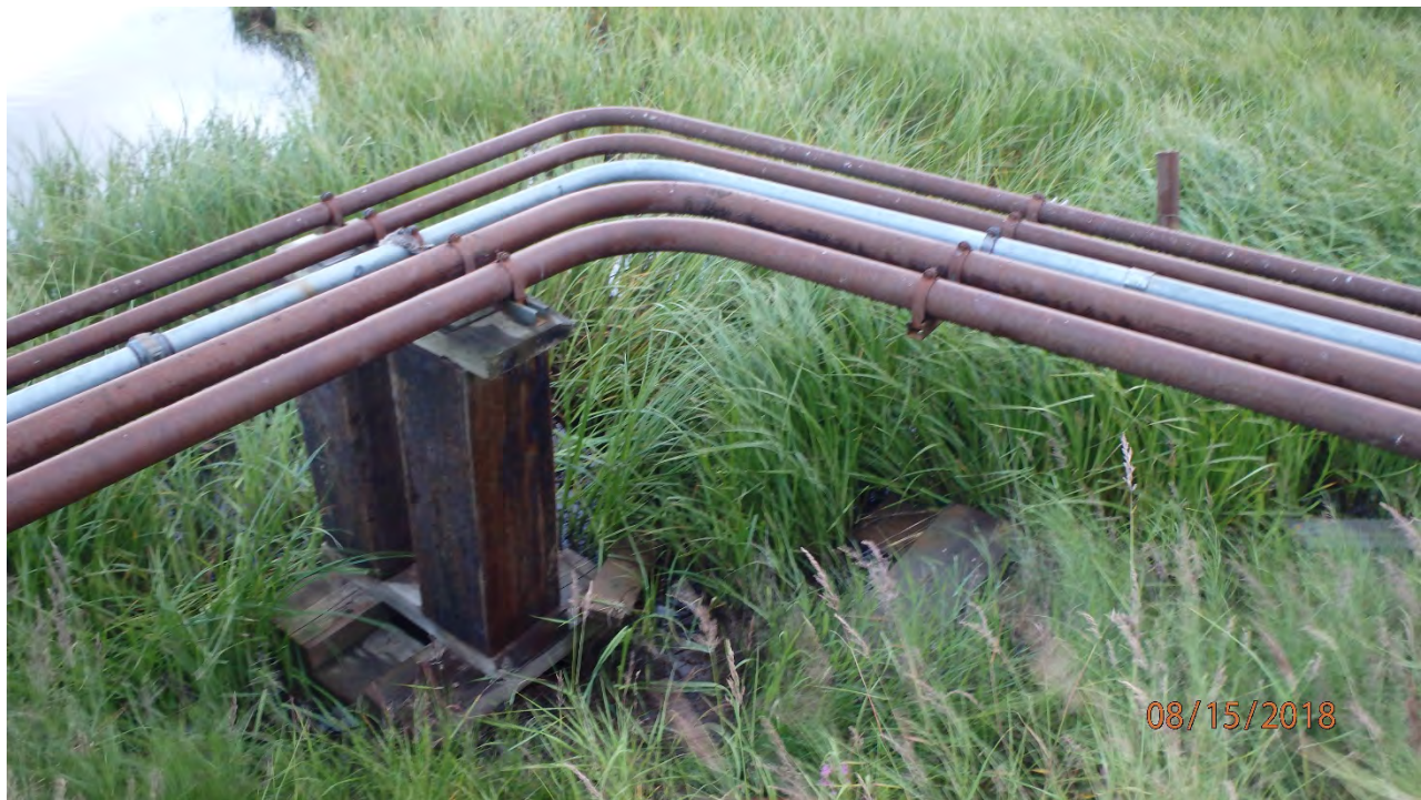
FIGURE 17: PIPE IS SUPPORTED ON UNSECURED CRIB PILES THAT HAVE FALLEN OVER IN SOME AREAS.
