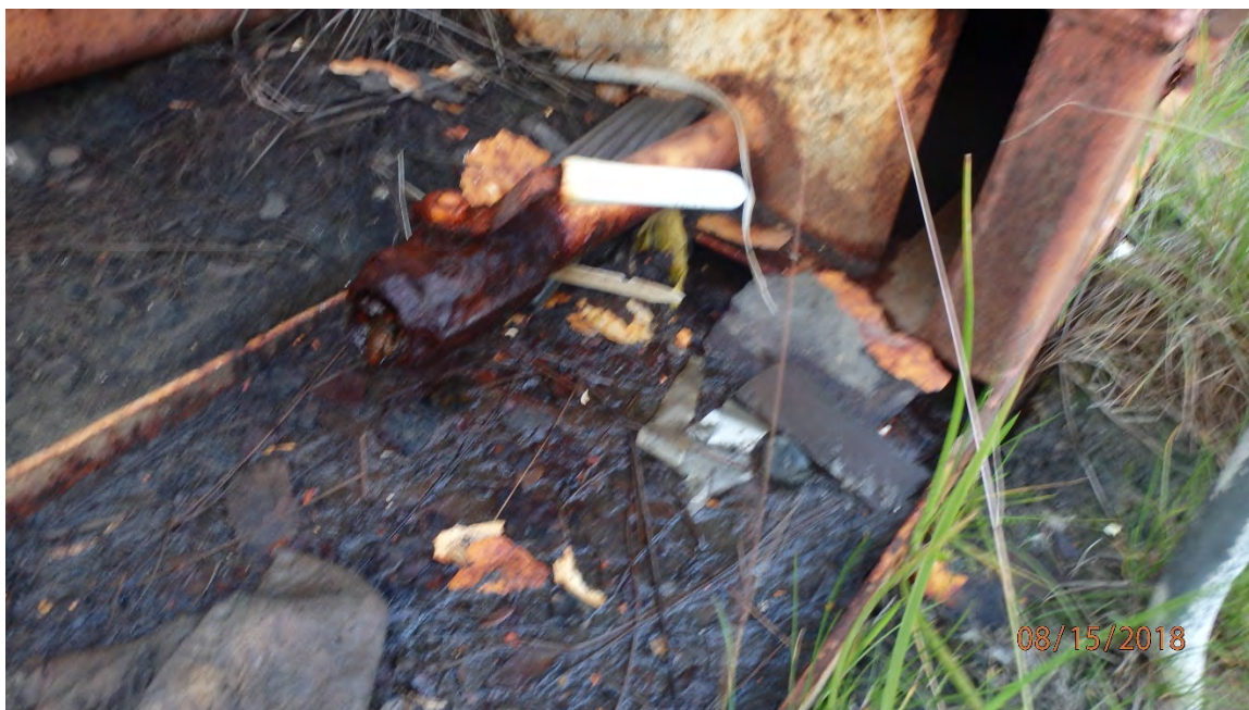
FIGURE 12: FAILED CONTAINMENT DRAIN VALVE FOR DISPENSER CABINET AT RIVER. VALVE WAS FOUND DRIPPING WATER DURING INSPECTION.
