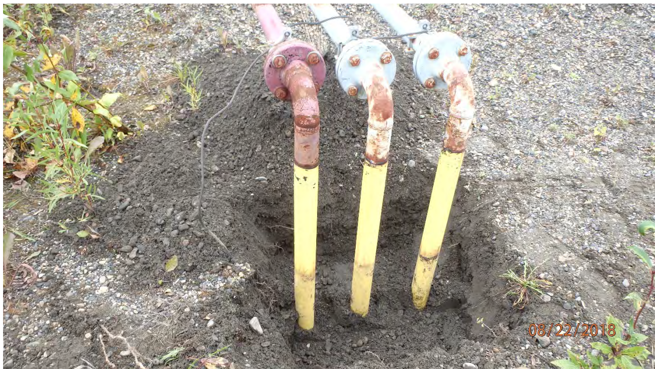
FIGURE 12: 2-INCH SERVICE LINE RISERS IN TANK FARM. GASOLINE ON LEFT, DIESEL (X2) ON RIGHT. 18-INCH DEEP EXCAVATION TO ASSESS COATING CONDITION.
