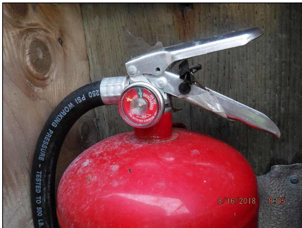
Photograph 7: Looking at undercharged fire extinguisher.
