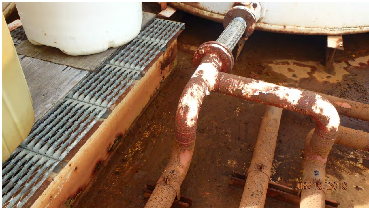
FIGURE 19: CROSS OVER TO FOUR ABANDONED VERTICAL TANKS. NO ISOLATION VALVES UNTIL TANK NOZZLES. 1 LARGE DEAD-LEG.
