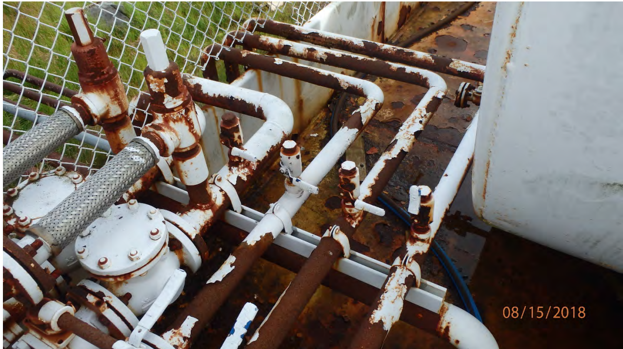
FIGURE 18: CARGO AND SERVICE PIPING CONDITION AS IT ENTERS CONTAINMENT. NOTE HIGH POINT VENT FOR LINE ON RIGHT (COUNCIL TANK AND WINTER DISPENSER) IS SEIZED IN THE OPEN POSITION.
