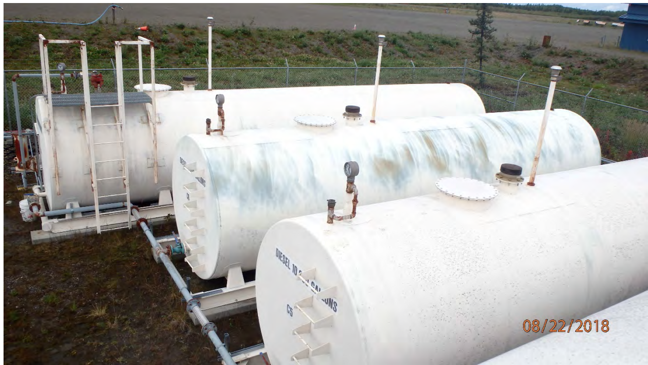
FIGURE 5: REFURBISHED TANKS SHOWING COATINGS FAILURES DUE TO UV DEGRADATION
