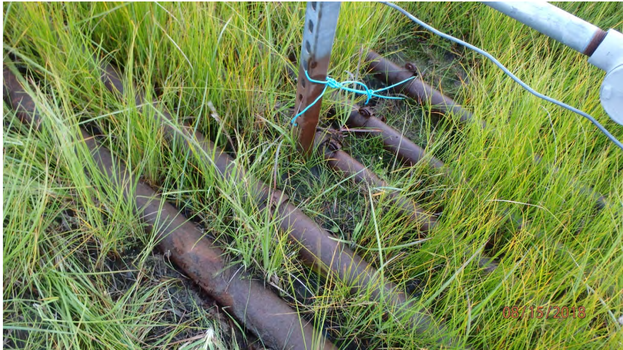
FIGURE 16: TYPICAL CARGO AND SERVICE LINE CONDITION IN LOW AREA, IN CONTACT WITH SOIL/WATER, SOME PIPE CLAMPS COMPLETELY CORRODED.
