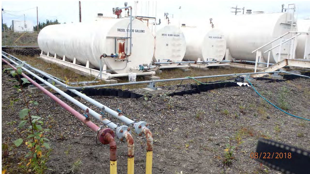
FIGURE 1: THREE REFURBISHED DIESEL TANKS FROM THE ORIGINAL TANK FARM (C5, C6 AND S1)
