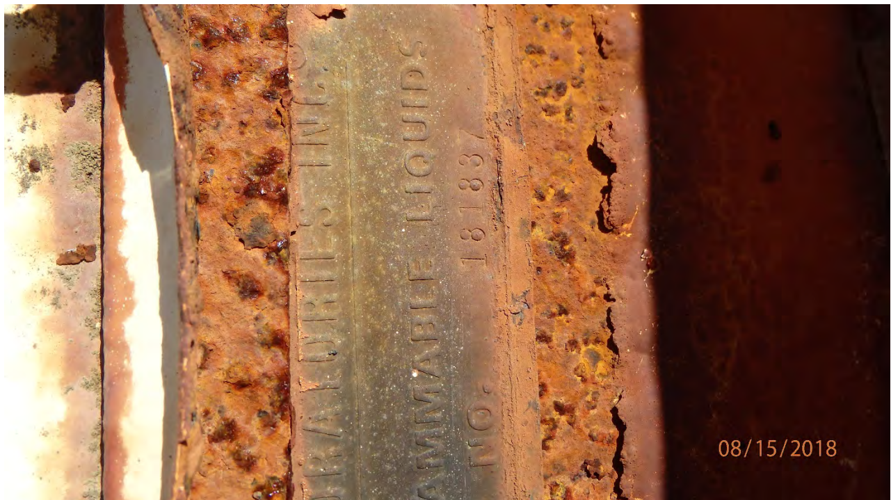
FIGURE 10: UL LISTING FOR TANK 1. THIS IS THE ONLY TANK WITH ANY LISTING INFORMATION.
