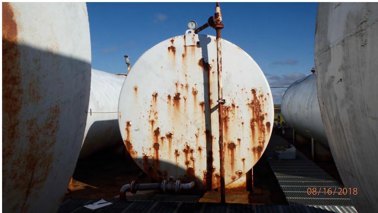
FIGURE 3: TANK 3 HEAD AND PIPING, TYPICAL CONDITION.
