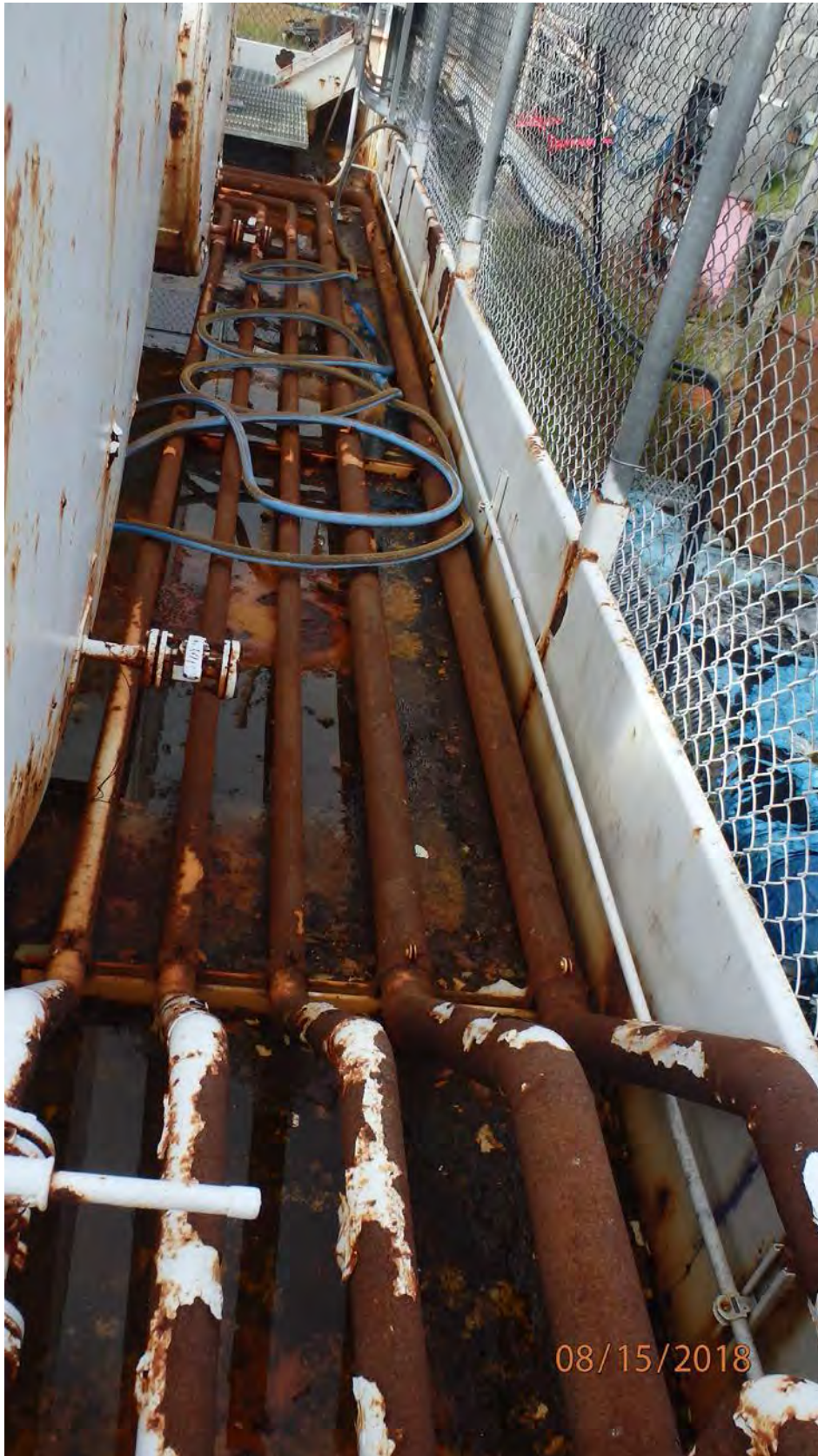
Typical tankfarm piping condition showing complete coating failure and generalized corrosion.
