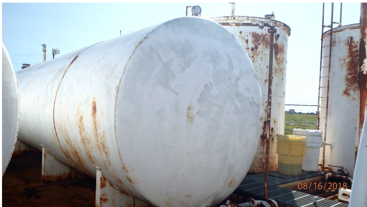
FIGURE 6: TYPICAL SHELL AND ELLIPTICAL HEAD COATING CONDITION FOR TANKS 10, 11 AND 12. 23,000 GALLONS EACH.
