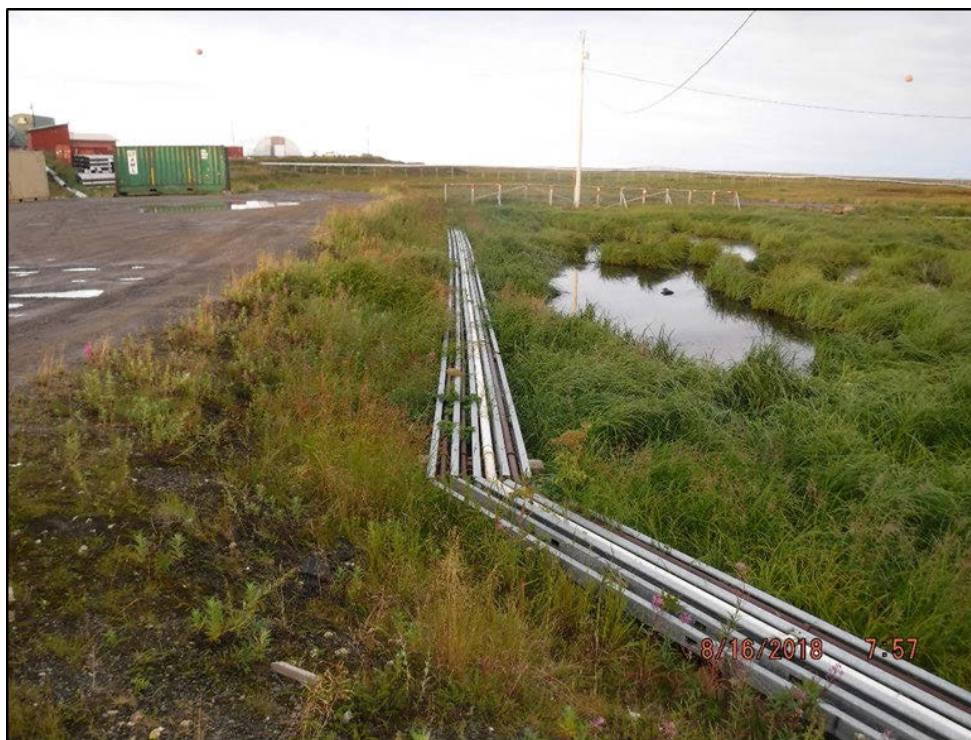
Photograph 3: Looking south along pipe run. Note retrofitted metal framing stud armoring.
