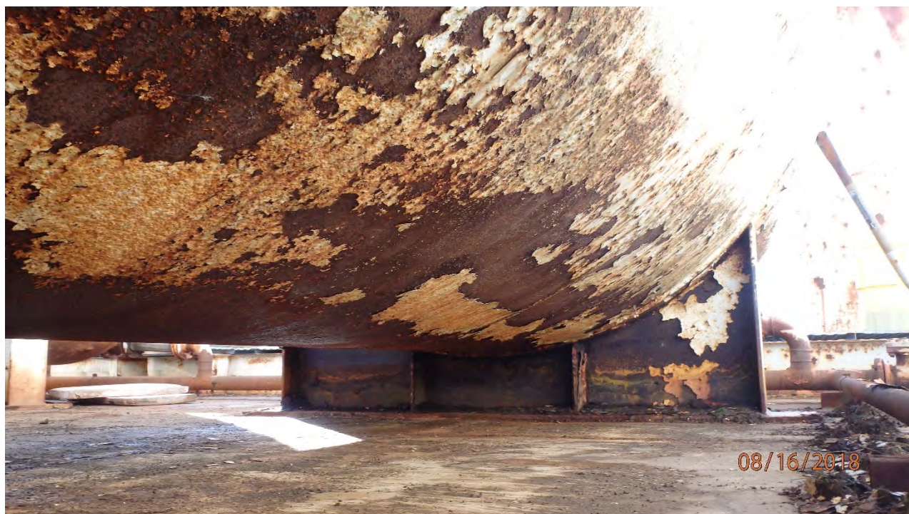
FIGURE 4: TYPICAL COATING CONDITION FOR THE BOTTOM 4 TO 8 FEET OF ALL TANK SHELLS. ALL TANKS SHOW SOME DEGREE OF CORROSION IN THIS AREA WITH TANK 4 EXHIBITING THE WORST PITTING AND GENERAL WALL LOSS.
