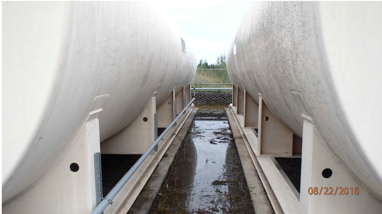
FIGURE 9: TYPICAL TANK SUPPORTS AND CONCRETE PIER FOUNDATIONS.
