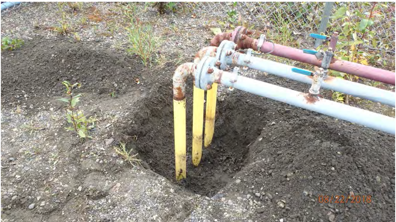
General piping condition with surface rust at all welded connections, elbows and flanges. Below grade yellow jacket in excellent condition.
