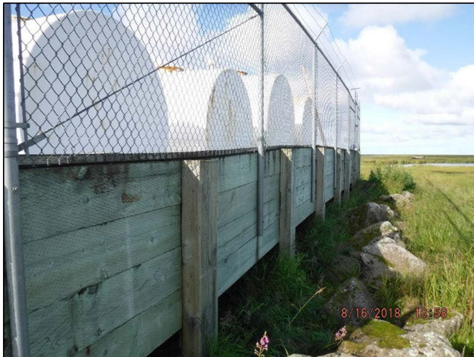
Photograph 22: Looking west along the north side of the tank containment wall. Note gap of exposed liner beneath lowest horizontal timber.
