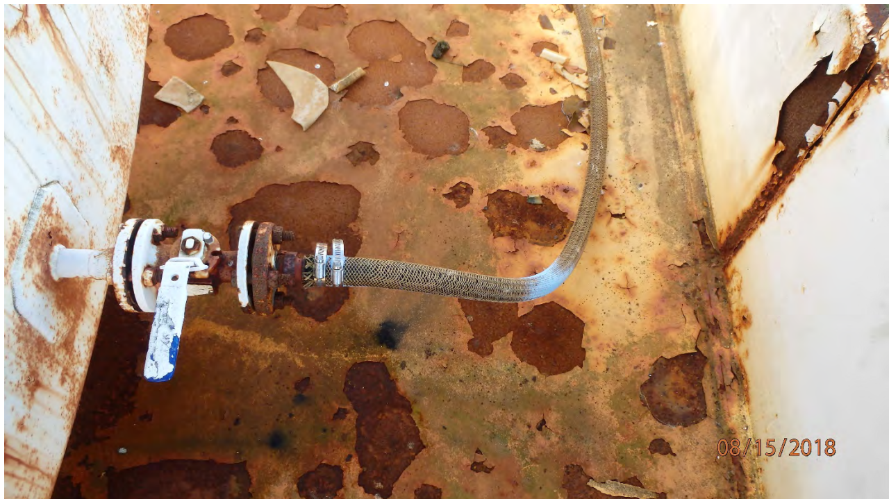
FIGURE 21: FUEL TRANSFER HOSE CONNECTED TO WATER-DRAW NOZZLE ON TANK 5. NO LOCK ON VALVE AND HOSE TERMINATES OUTSIDE OF CONTAINMENT IN OLD DISPENSER SHACK. NOTE UV DEGRADATION OF RUBBER.
