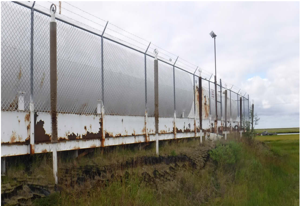
Figure 3: Pad slumping
