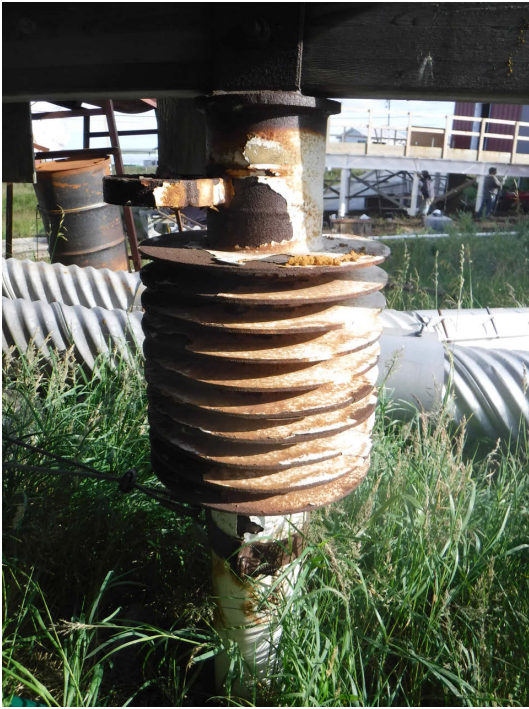
Figure 9: Corrosion, Old Power House
