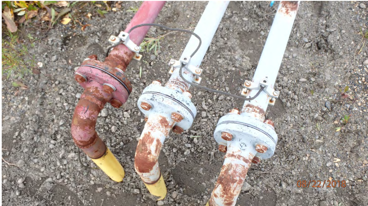
FIGURE 11: 2-INCH SERVICE LINE RISERS IN TANK FARM. GASOLINE ON LEFT, DIESEL (X2) ON RIGHT. GROUNDING ROD CONNECTED TO TANK FARM SIDE OF ISOLATION FLANGES.
