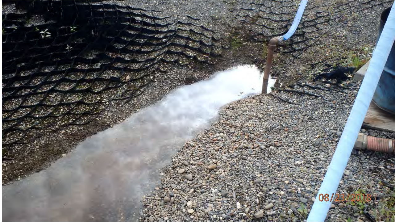
FIGURE 21: CATCHMENT ADJACENT TO AIRCRAFT HEADER AND DIESEL DISPENSER. FUEL SHEEN ON WATER.
