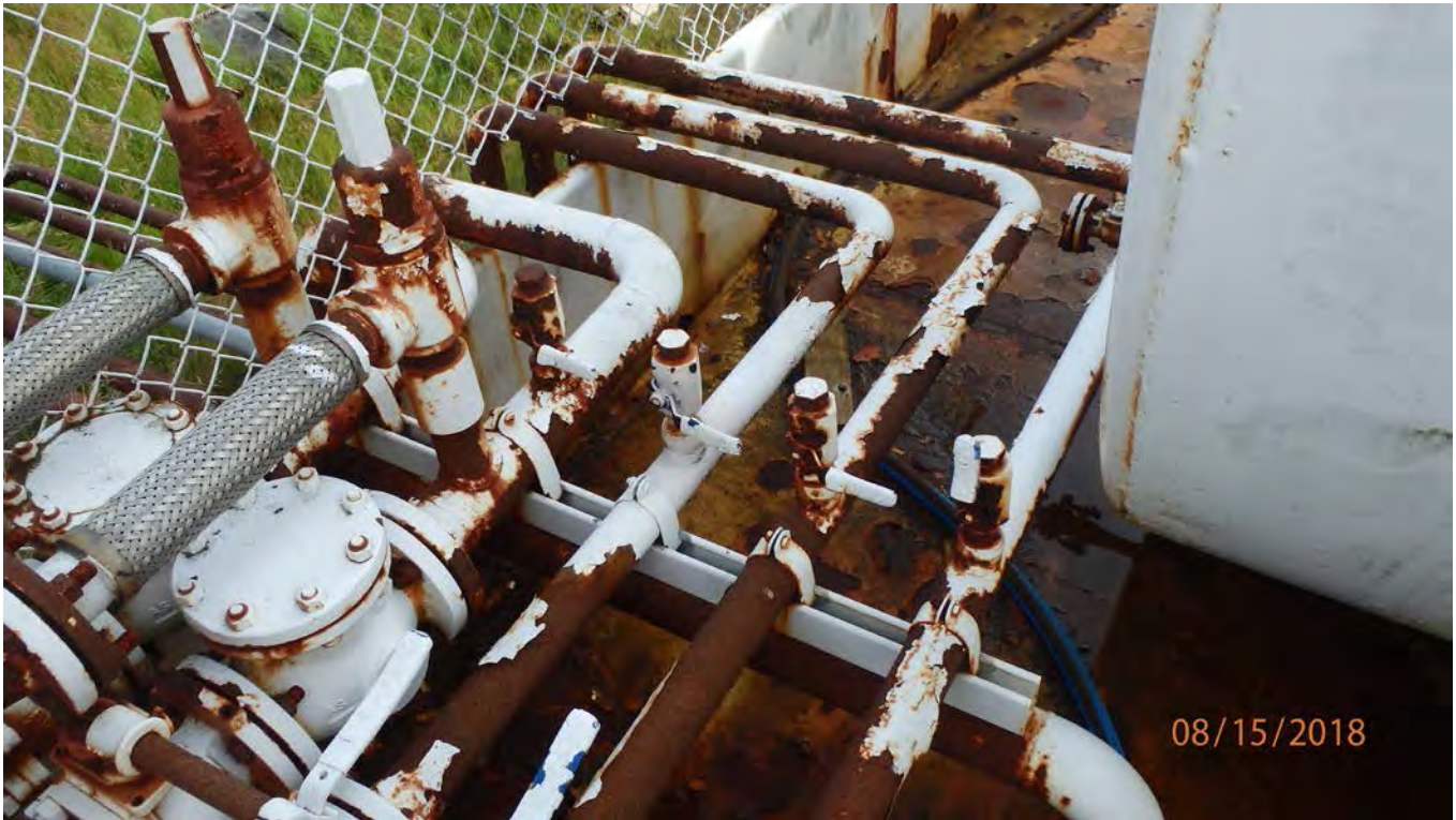
Cargo and service lines at tank farm wall. Highpoint vent valve on 2-inch line to Council tank is corroded in the open position
