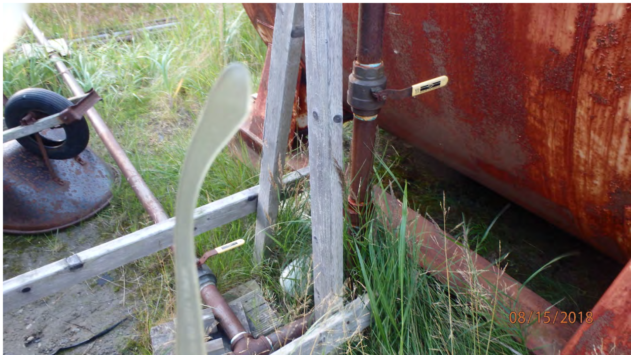
FIGURE 23: 2 BRASS VALVES IN FUEL SERVICE AT SECONDARY DISPENSER AND COUNCIL TANK.
