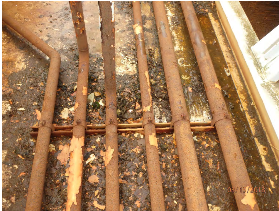
FIGURE 20: TYPICAL PIPING CONDITION IN TANK FARM. PIPING WAS PARTIALLY SUBMERGED ON ARRIVAL. PIPING IS CLAMPED TO UNI-STRUT WHICH IS WELDED TO THE FLOOR OF CONTAINMENT.
