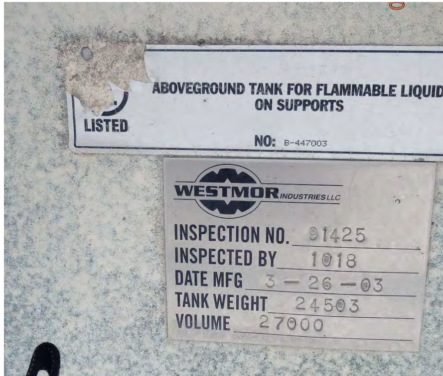
FIGURE 6: UL LISTING INFORMATION FOR TANK C1, GASOLINE STORAGE TANK
