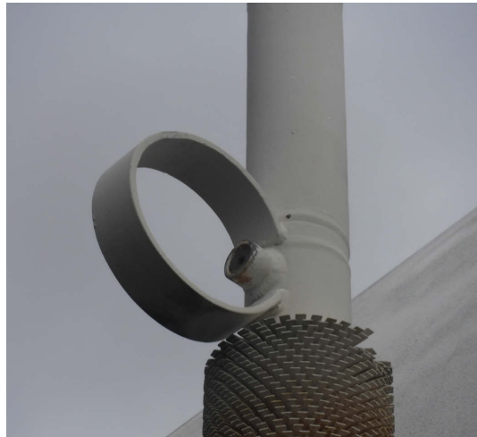
Figure 5: Missing valve on Unit #7
