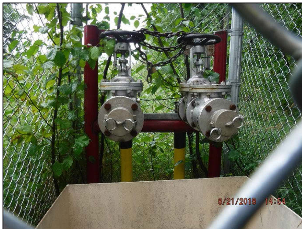
Photograph 10: Marine header.
