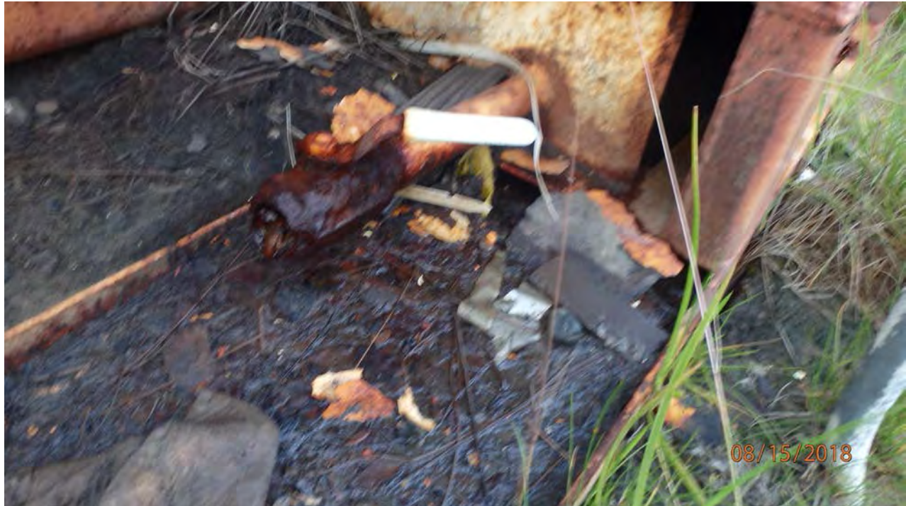
Dispenser containment drain valve found failed and leaking.
