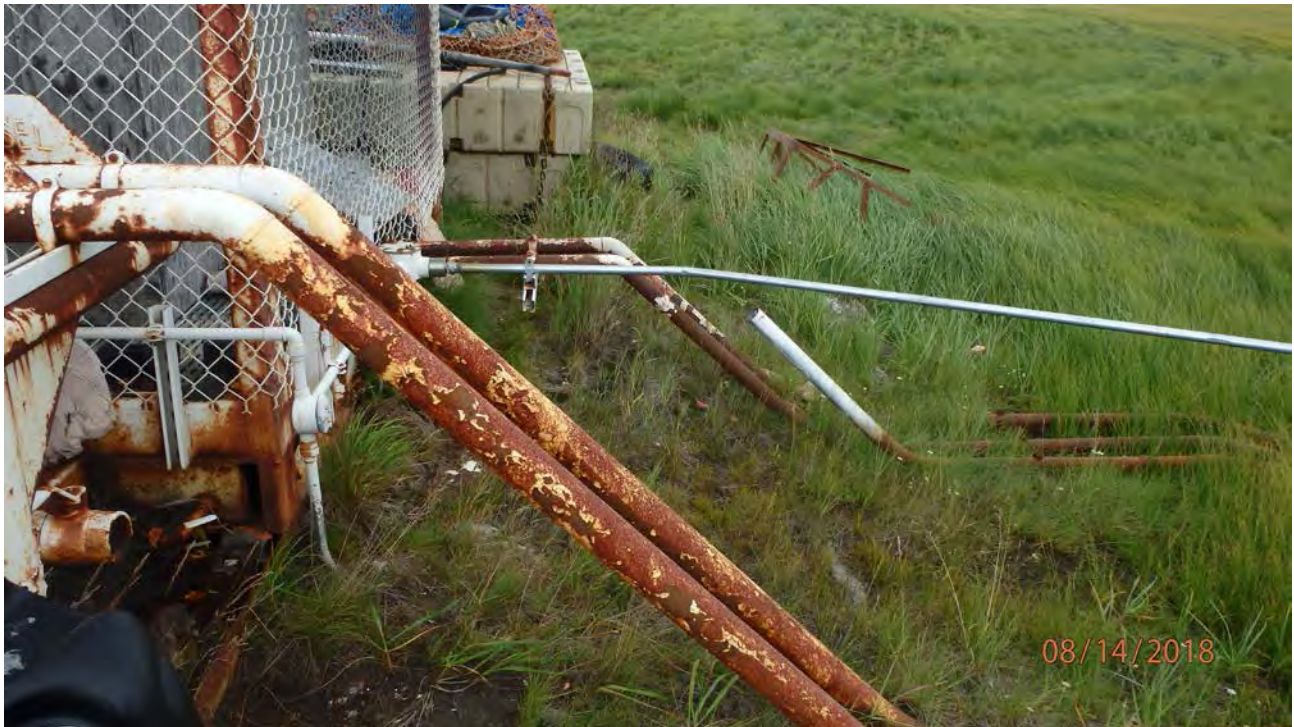
Cargo and service piping at dispenser transitioning to on grade.
