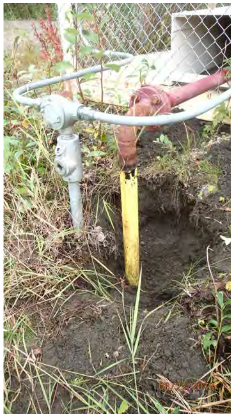
Coating condition at gasoline dispenser transition.
