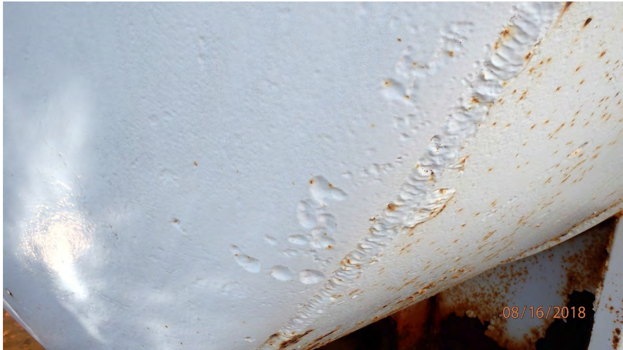
FIGURE 7: TYPICAL ISOLATED PITTING ON THE ELLIPTICAL HEADS FOR TANKS 10-12. MAXIMUM DEPTH 100 MILS
