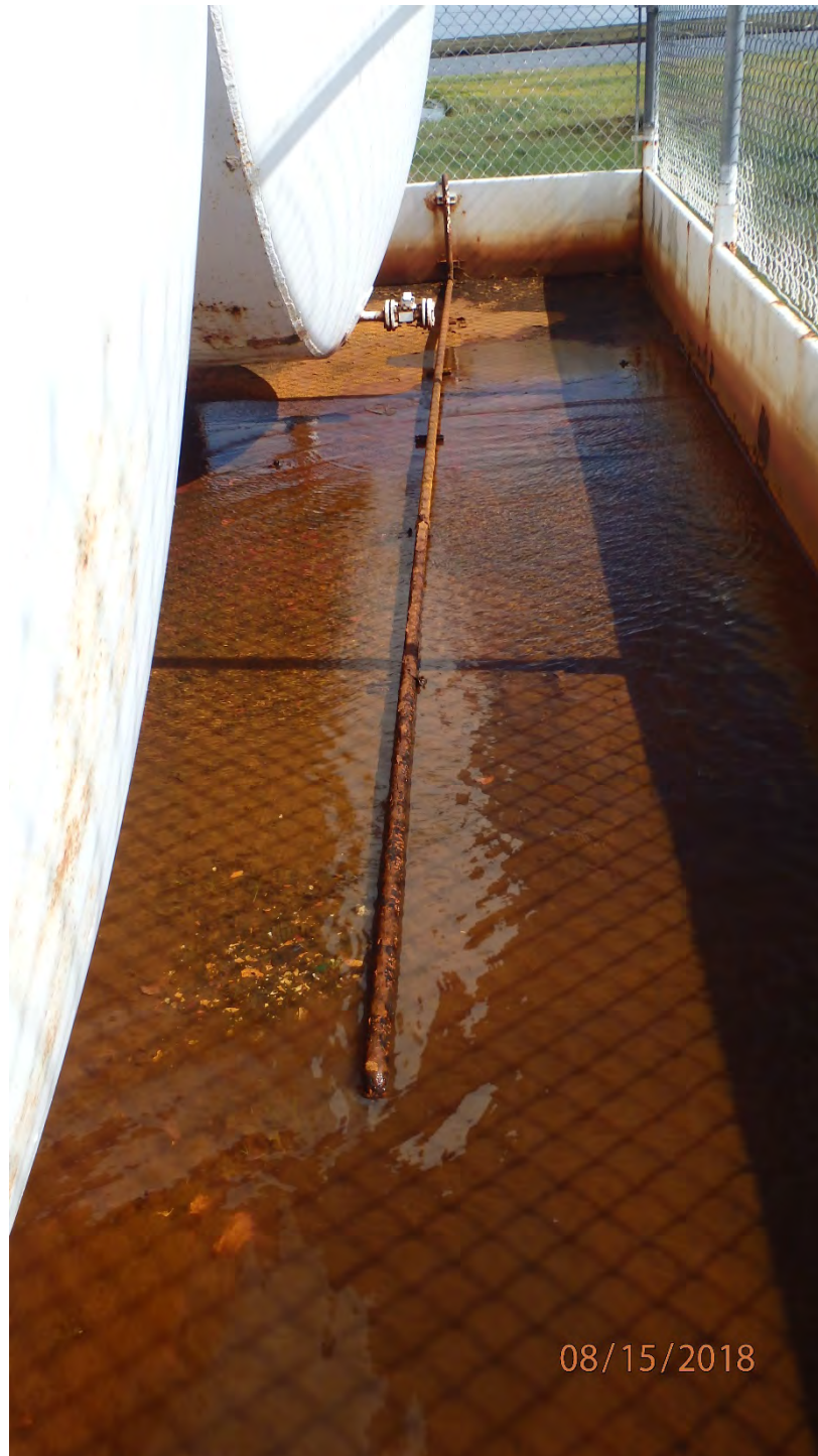
FIGURE 24: ONE OF THREE DRAIN SUMPS FOR CONTAINMENT. SUMPS ARE 10-INCH DIA WITH ELLIPTICAL HEADS. ALL THREE SUMPS WERE FOUND FILLED WITH SCALE AND DEBRIS AND WITH GENERAL WALL LOSS DUE TO CORROSION.
