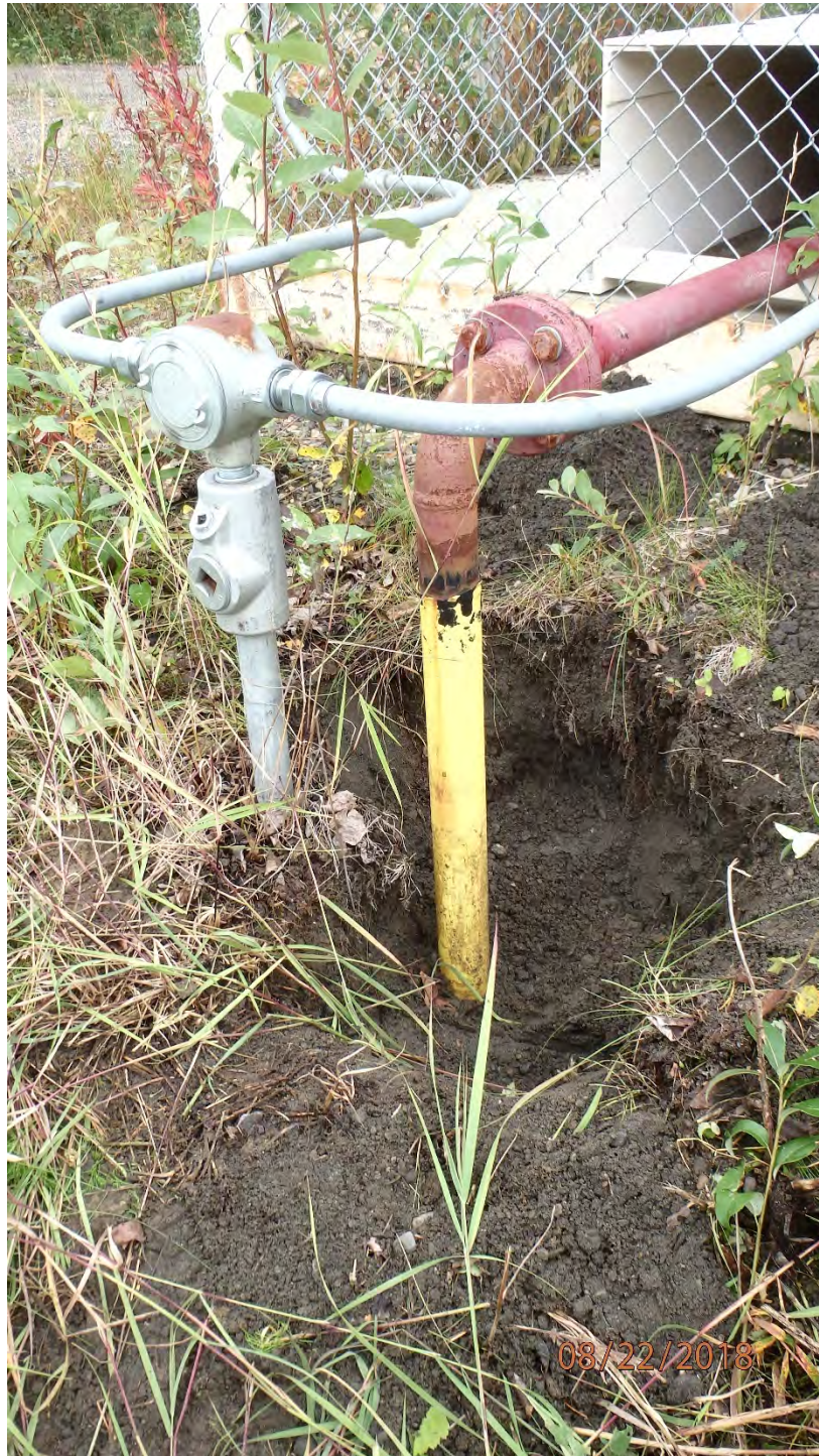
FIGURE 15: GASOLINE DISPENSER RISER 18-INCH DEEP EXCAVATION. COATING IN EXCELLENT CONDITION.
