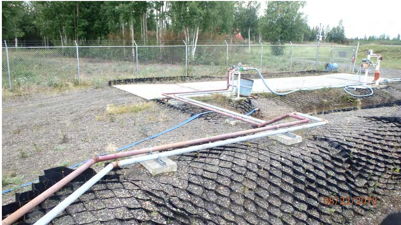
FIGURE 18: HEADER PIPING AT TRUCK RACK. NOTE FUEL HOSE FOR OFFLOADING AIRCRAFT IS LEFT ATTACHED AND EXPOSED BETWEEN FUEL DELIVERIES. NOTE GEOGRID FORMWORK IS EXPOSED.
