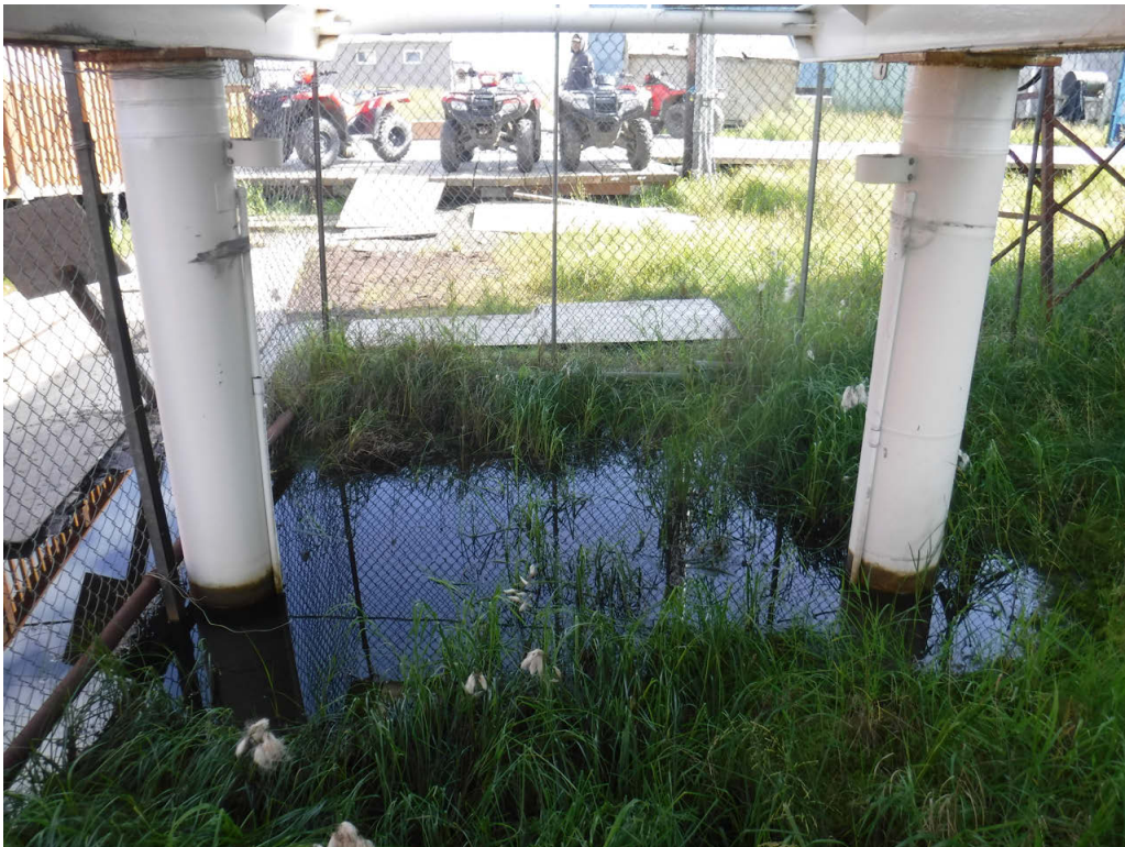
Figure 11: Extensive ponded water around piles under fuel tank at New Power House
