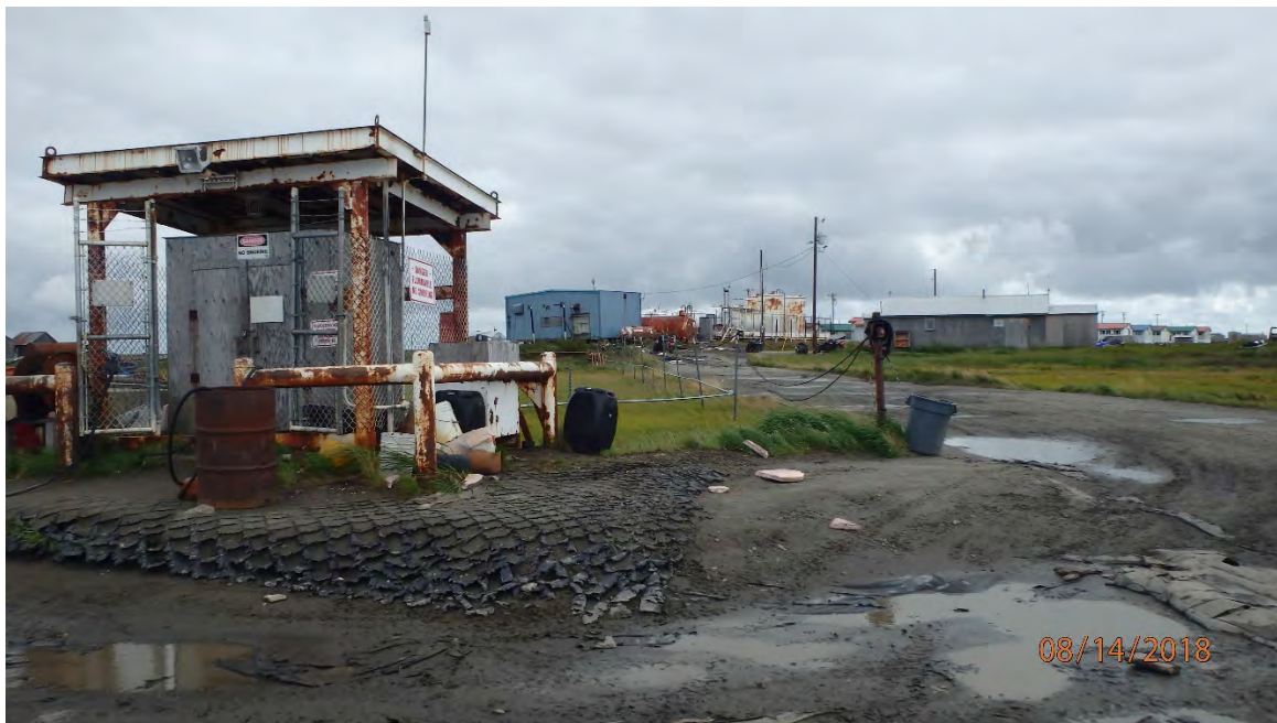
FIGURE 11: 3-INCH BARGE HEADER RISERS AT RIVER, ADJACENT TO FUEL DISPENSER. OLD POWER PLANT AND MARINA TANK FARM IN BACKGROUND.
