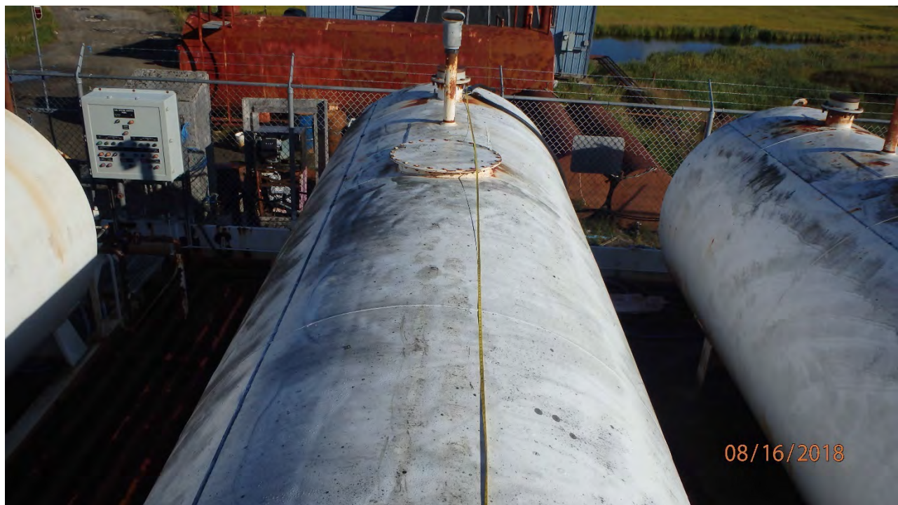
FIGURE 2: TYPICAL CONDITION TOP OF TANKS, TANK 2 THROUGH 5. 10,000 GALLONS EACH.
