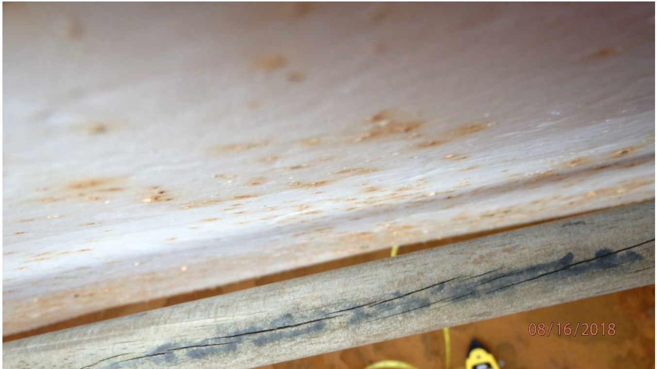
FIGURE 9: DENTING PRESENT IN SHELL FOR TANK 12. MAX DEFORMATION IS .75-INCHES FOR A DENT 7 FEET LONG BY 3.5 FEET CIRCUMFERENTIALLY. FIVE ADDITIONAL SMALLER DIAMETER DENTS PRESENT ON THIS TANK.
