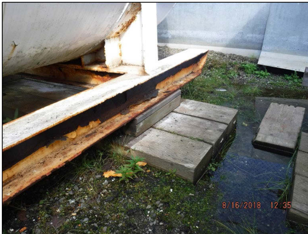
Photograph 20: Typical use of dimensional lumber used for cribbing on top of original treated wood foundation.
