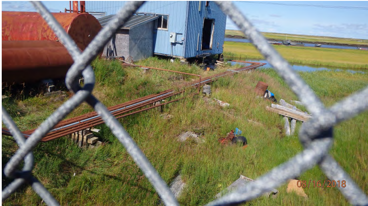
FIGURE 22: SERVICE LINE TO SECONDARY DISPENSER AND COUNCIL TANK ON THE RIGHT SIDE OF PIPE RUN. NOTE SAG BECAUSE PIPING IS OFF OF SUPPORT. OPERATOR WAS WORKING TO FIX THIS WHILE WE WERE ON SITE.
