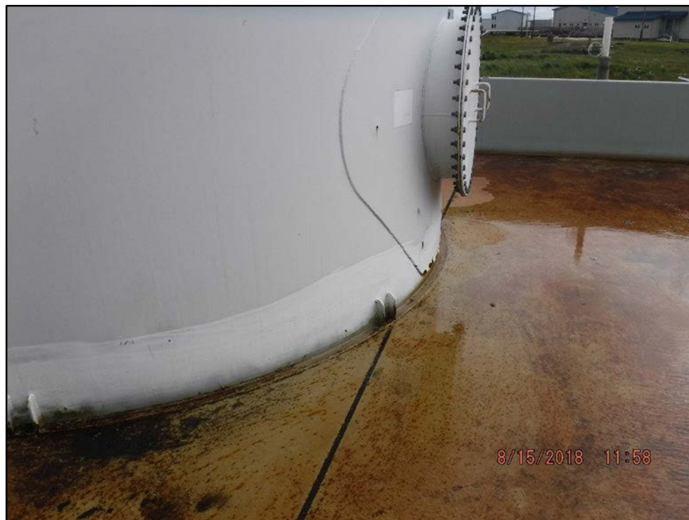
Photograph 4: Looking at standing water in containment and repainted tank bottom.
