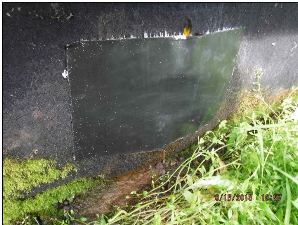
Photograph 19: Patched tear in liner material. Note water actively dripping.
