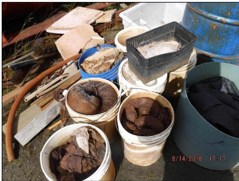
Photograph 10: Fuel saturated booms and sorbent pads outside of containment.
