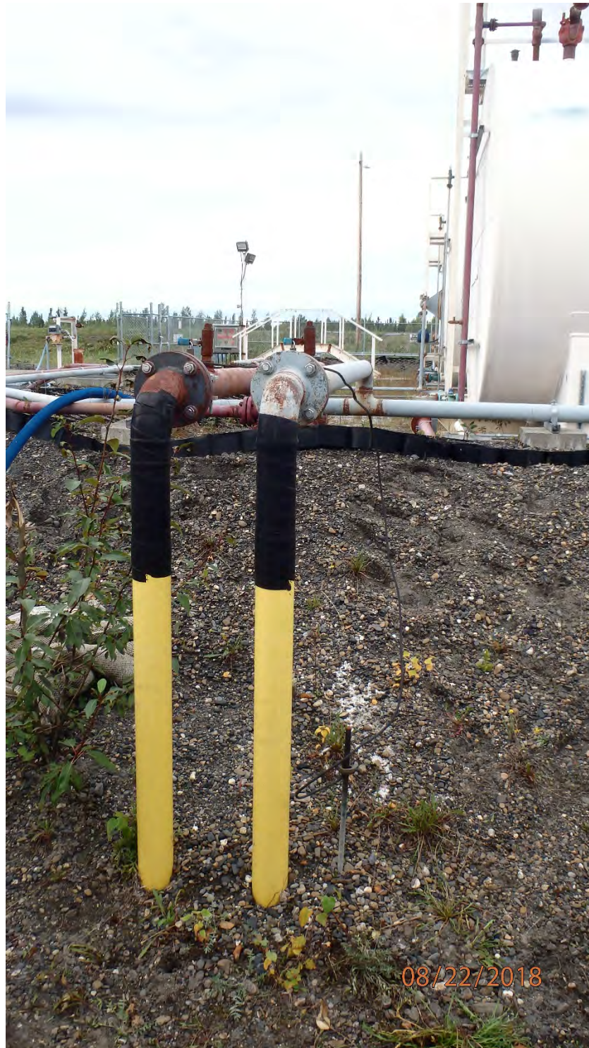
FIGURE 10: 3-INCH BARGE HEADER RISERS IN TANK FARM. GASOLINE ON LEFT, DIESEL ON RIGHT. GROUNDING ROD CONNECTED TO TANK FARM SIDE OF ISOLATION FLANGES.
