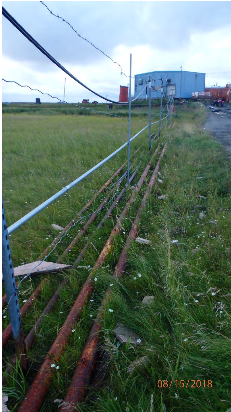
FIGURE 13: ~190 FEET OF CARGO AND SERVICE PIPING ON GRADE BETWEEN DISPENSER AND OLD POWER PLANT.
