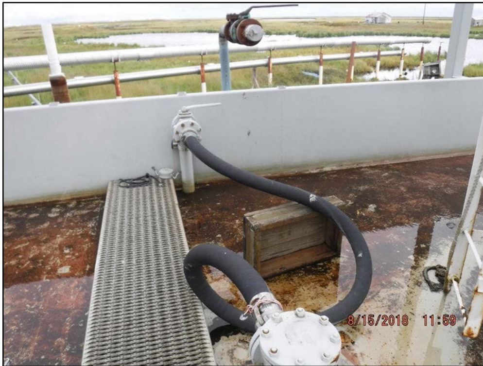
Photograph 3: Looking at marine header, school header, and rubber jumper line.
