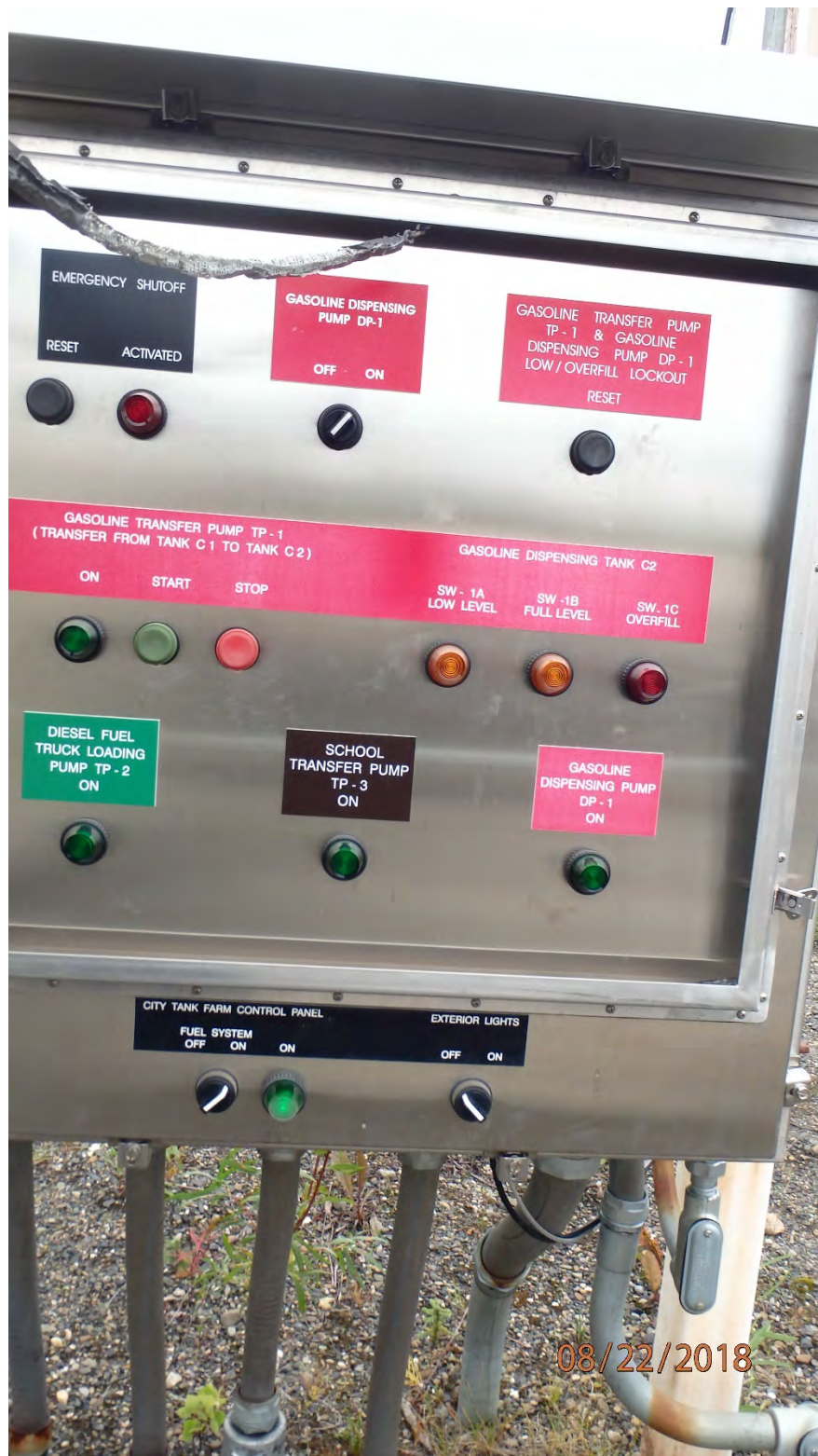
FIGURE 20: TANK FARM CONTROL PANEL.
