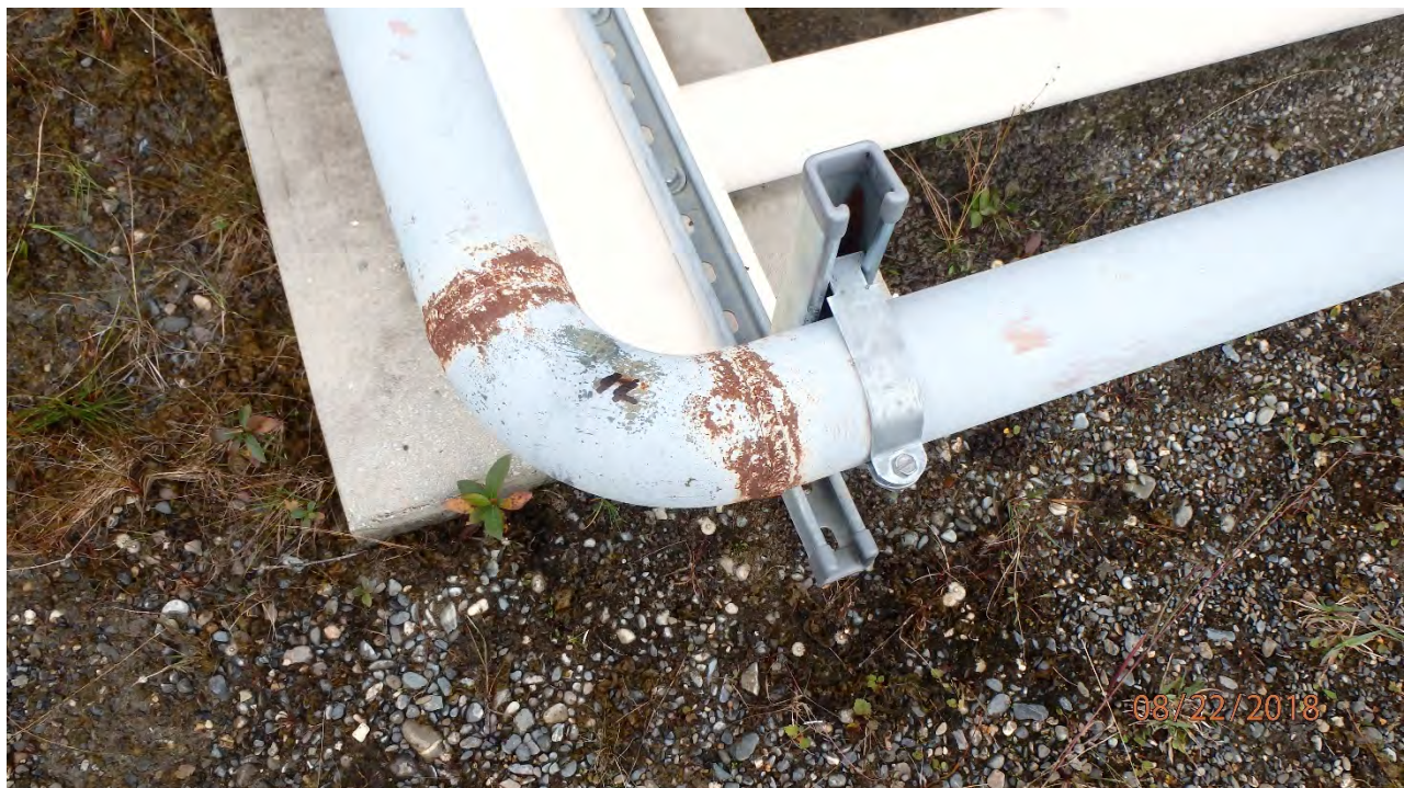
FIGURE 19: GALVANIZED UNI-STRUT AND PIPE CLAMP HANGERS/SUPPORTS. POSSIBILITY FOR DISSIMILAR METALS CORROSION IF PIPE COATINGS FAIL.
