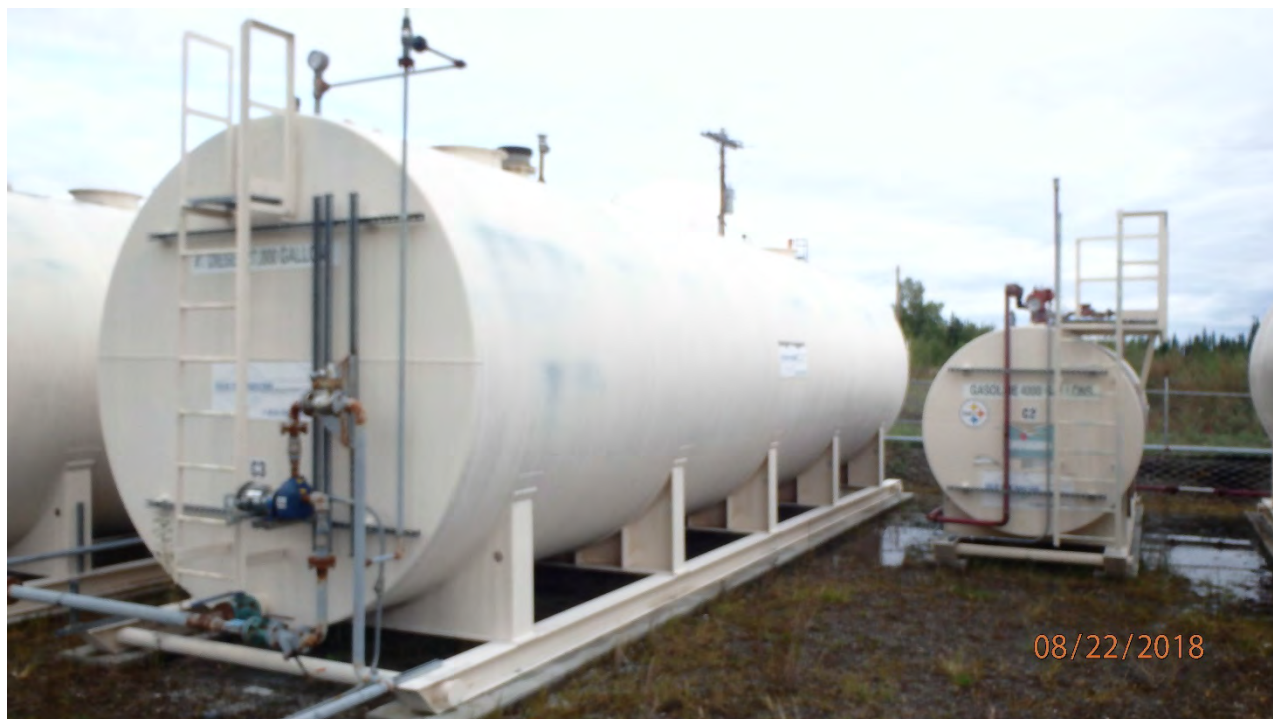
FIGURE 3: NEW DIESEL TANK LEFT (C3), NEW GASOLINE DISPENSING TANK RIGHT (C2)
