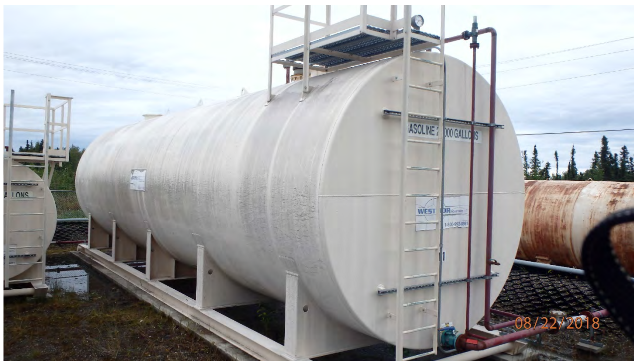
FIGURE 4: NEW GASOLINE DISPENSING TANK RIGHT (C1), CONTINGENCY TANK IN BACKGROUND.
