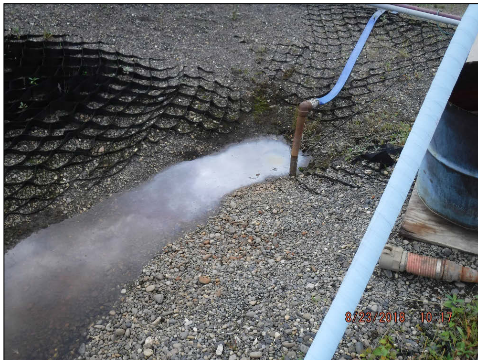
Photograph 12: Petroleum sheen seen within dike by fueling header on 23 August 2018.
